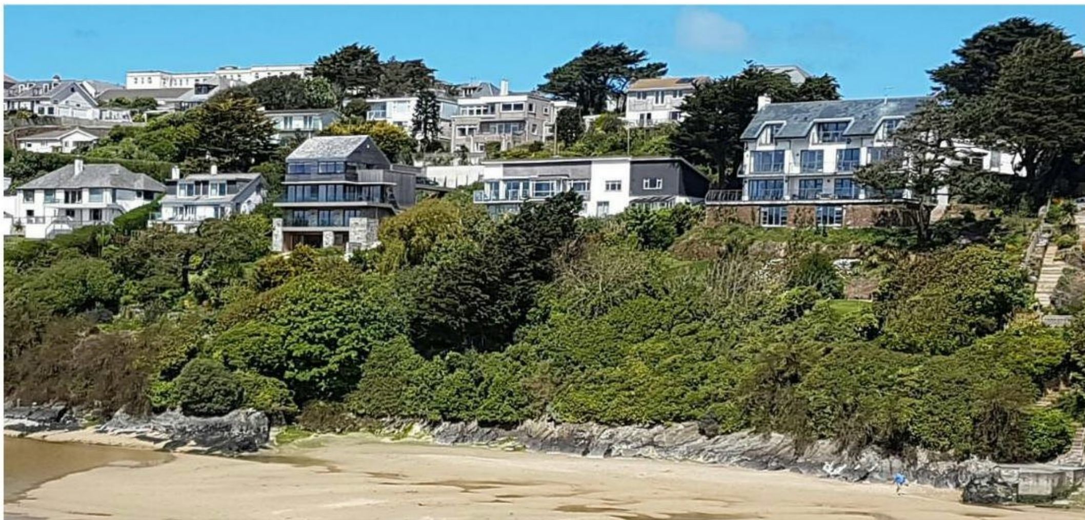
Existing View From The Gannel (South-East) Showing the large gap between Pine Hollow and Riverside
