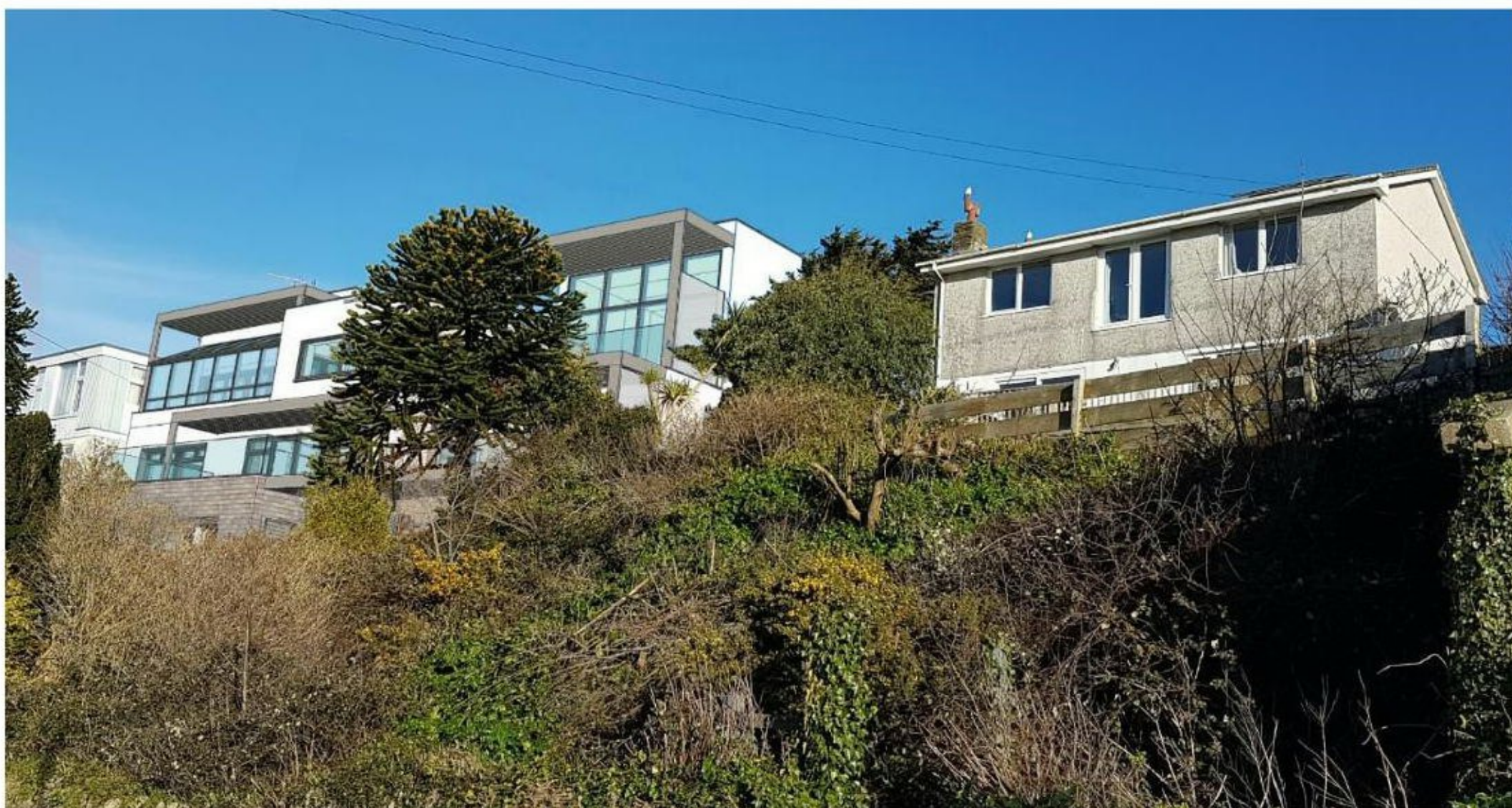
Proposed View From Riverside Avenue (South) Showing the Annex screened by retained mature planting and reading as 'one dwelling' with the rest of Pine Hollow that is overclad in the same materials
