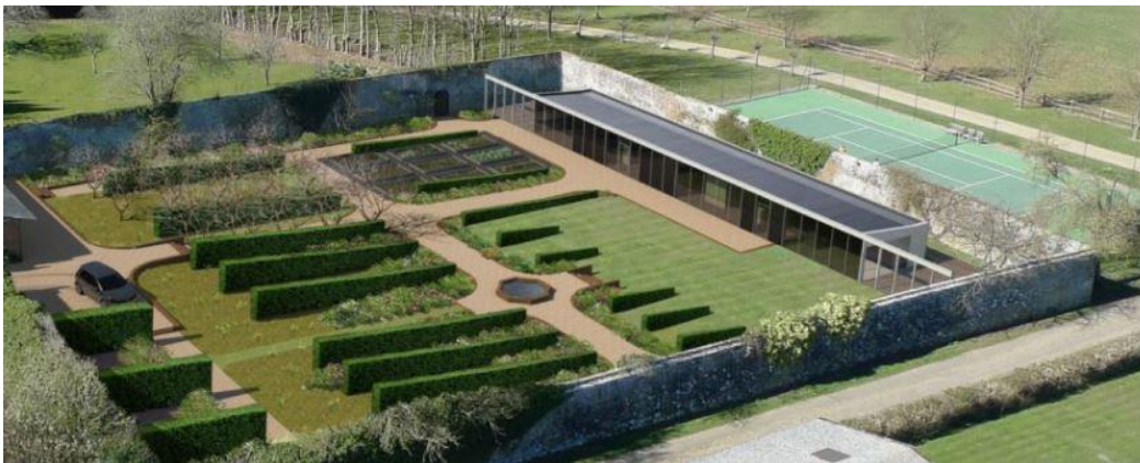
Figure 13 – Example of low level house within an existing walled garden with ridge sitting lower than the top of the garden wall.
