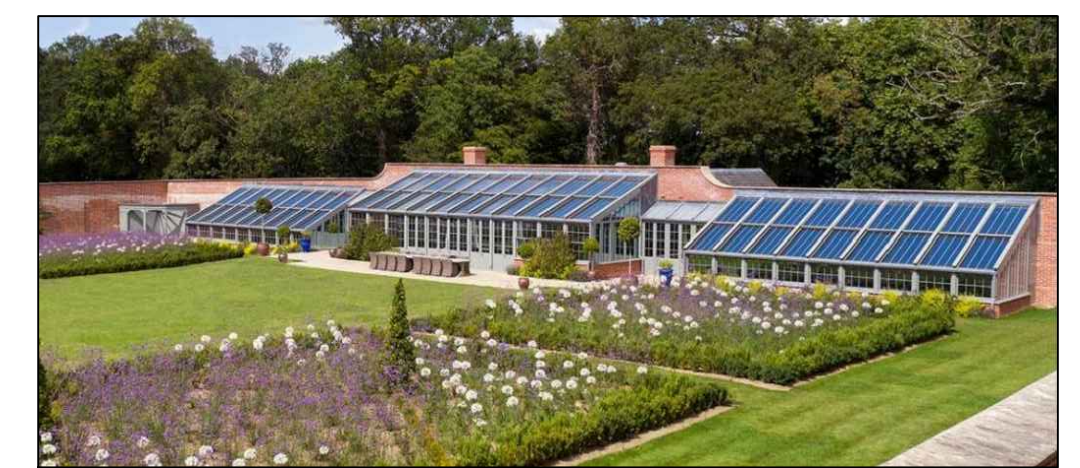
LARGE AREAS OF GLAZING TO MAXIMUM VIEWS AND LIGHT TO THE SOUTH
