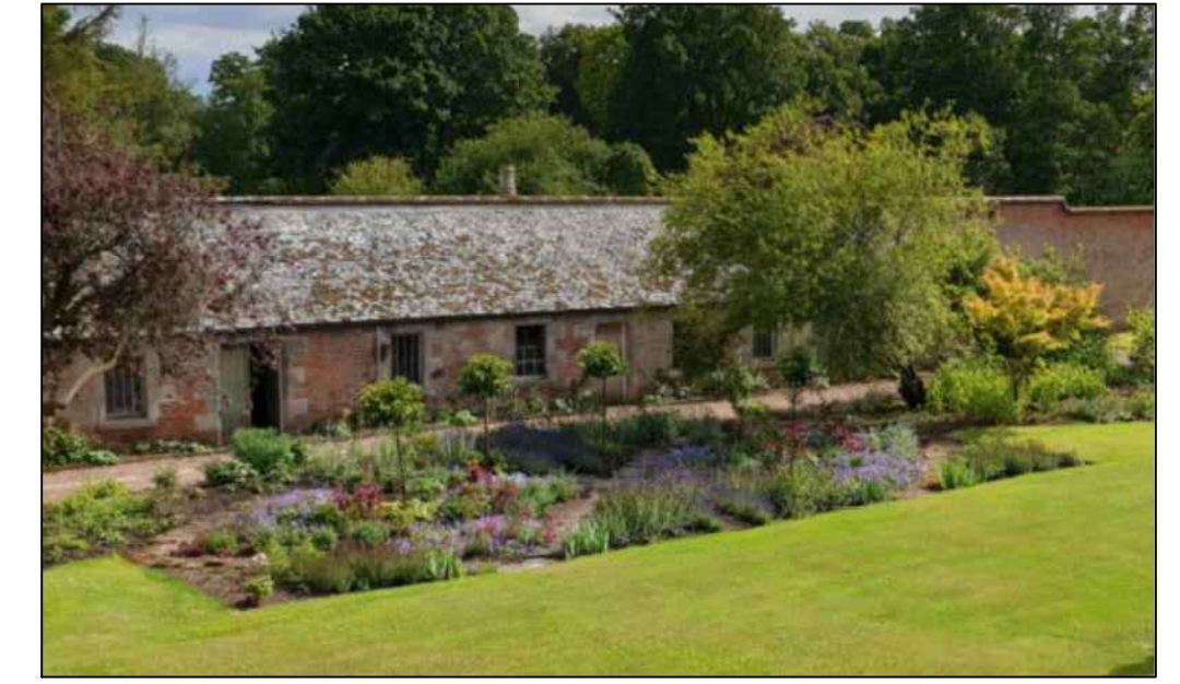
USE OF NATURAL STONE TO BLEND WITH STONE OF GARDEN WALLS & RIDGE HEIGHT OF HOUSE LOWER THAN TOP OF GARDEN WALL
