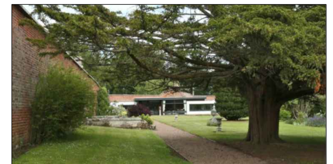
SIMPLE CONTEMPORARY BUILDING WITHIN TRADITIONAL WALLED GARDEN
