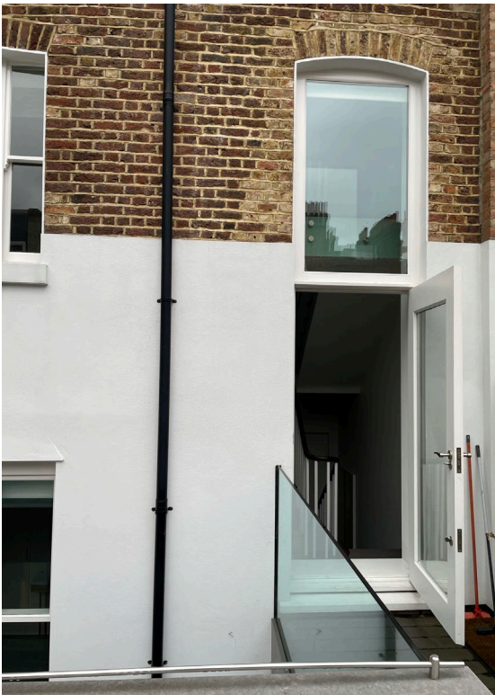
First Floor Terrace Access
