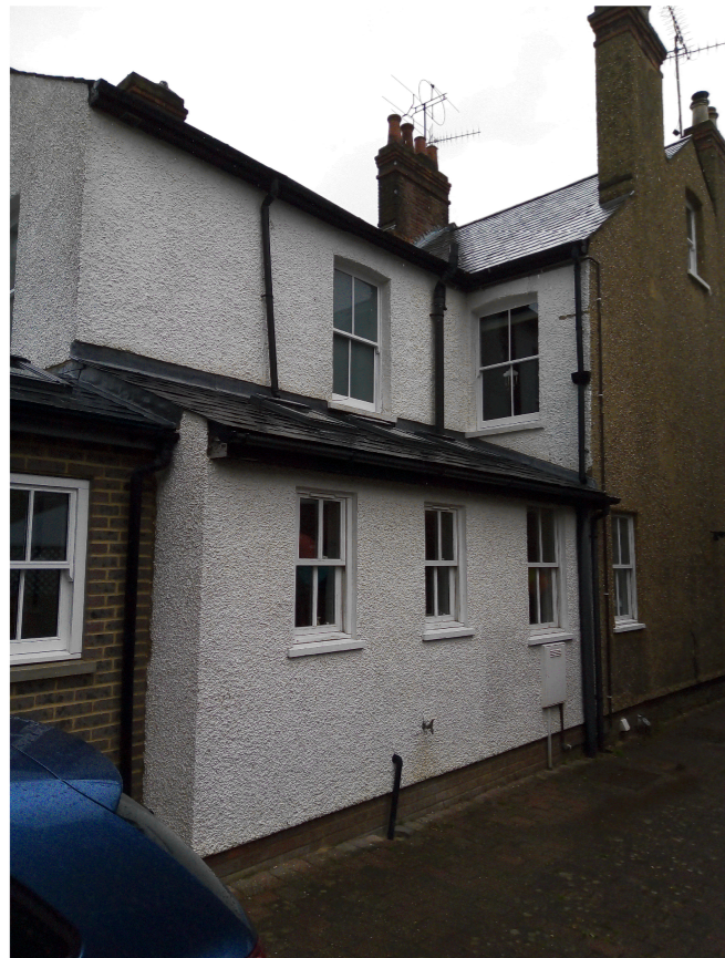
EXISTING REAR VIEW
