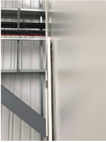
18 Gap to be finished.
