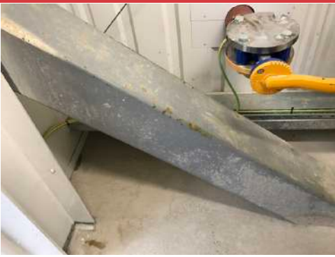
17 Steel work to be painted.
