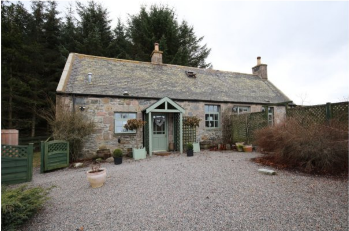
View of existing house from North
