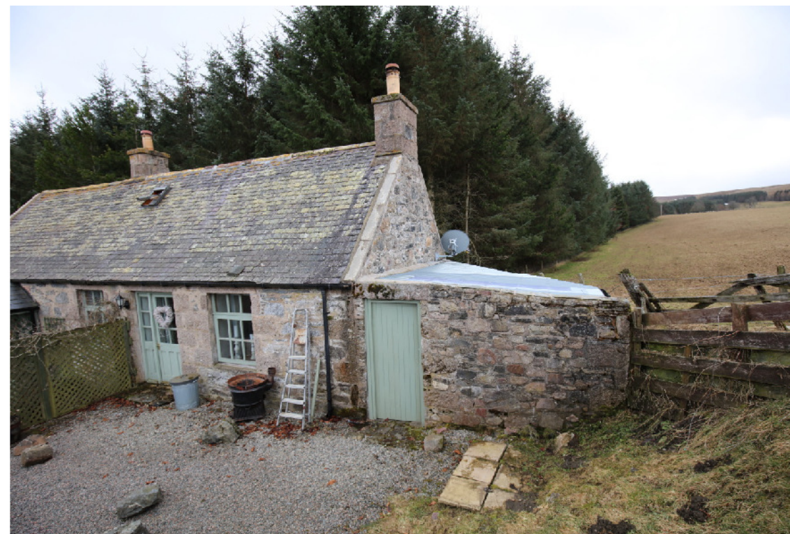
VIEW OF FRONT OF BUILDING FROM NORTH WEST OF SITE
