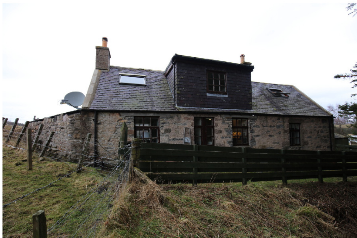
SOUTH ELEVATION OF HOUSE
