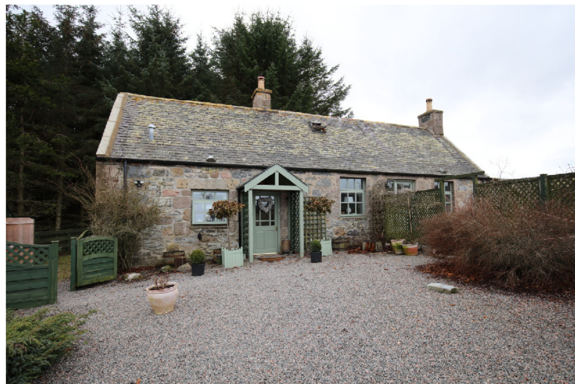
NORTH ELEVATION OF HOUSE
