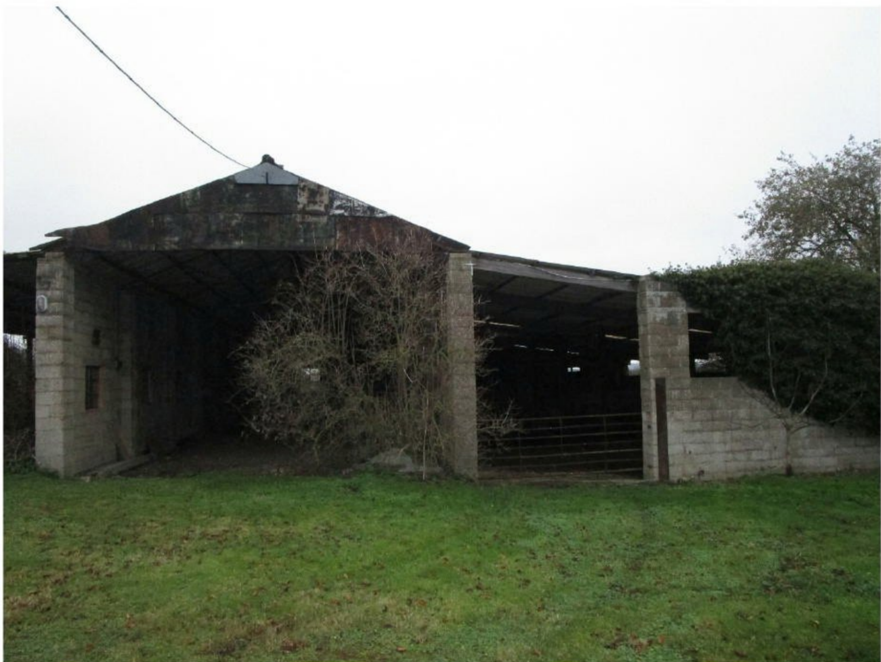
Figure 7 – the southern elevation view of both sections of the barn
