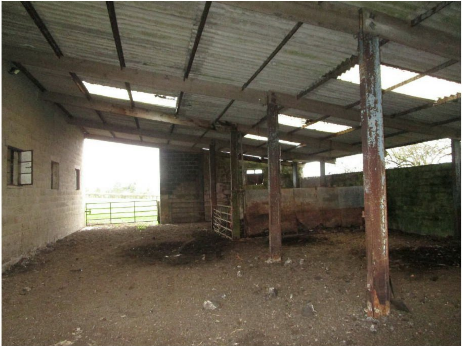
Figure 4 - the interior of the south-eastern lean-to section of the barn
