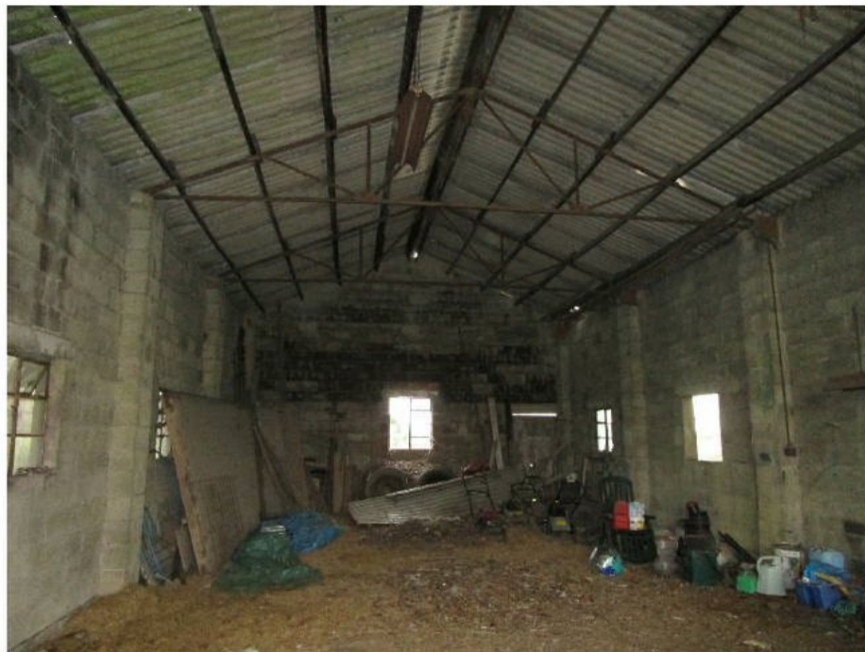
Figure 2 – The northern gable wall and side elevations of section one
