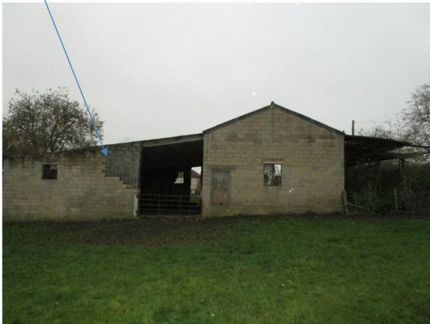
Figure 6 – the northern elevation
