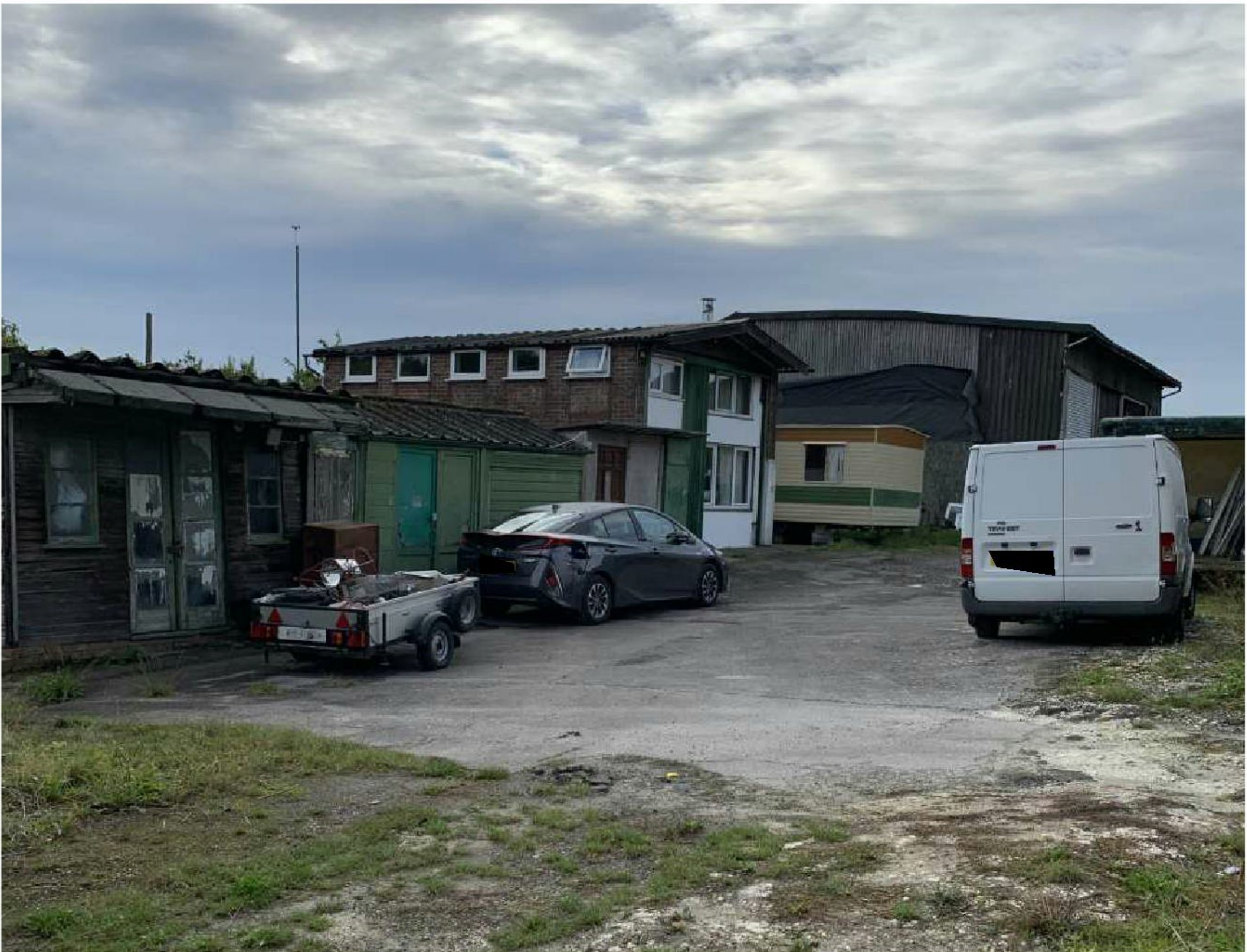
Workshop before fire and remodelling works
