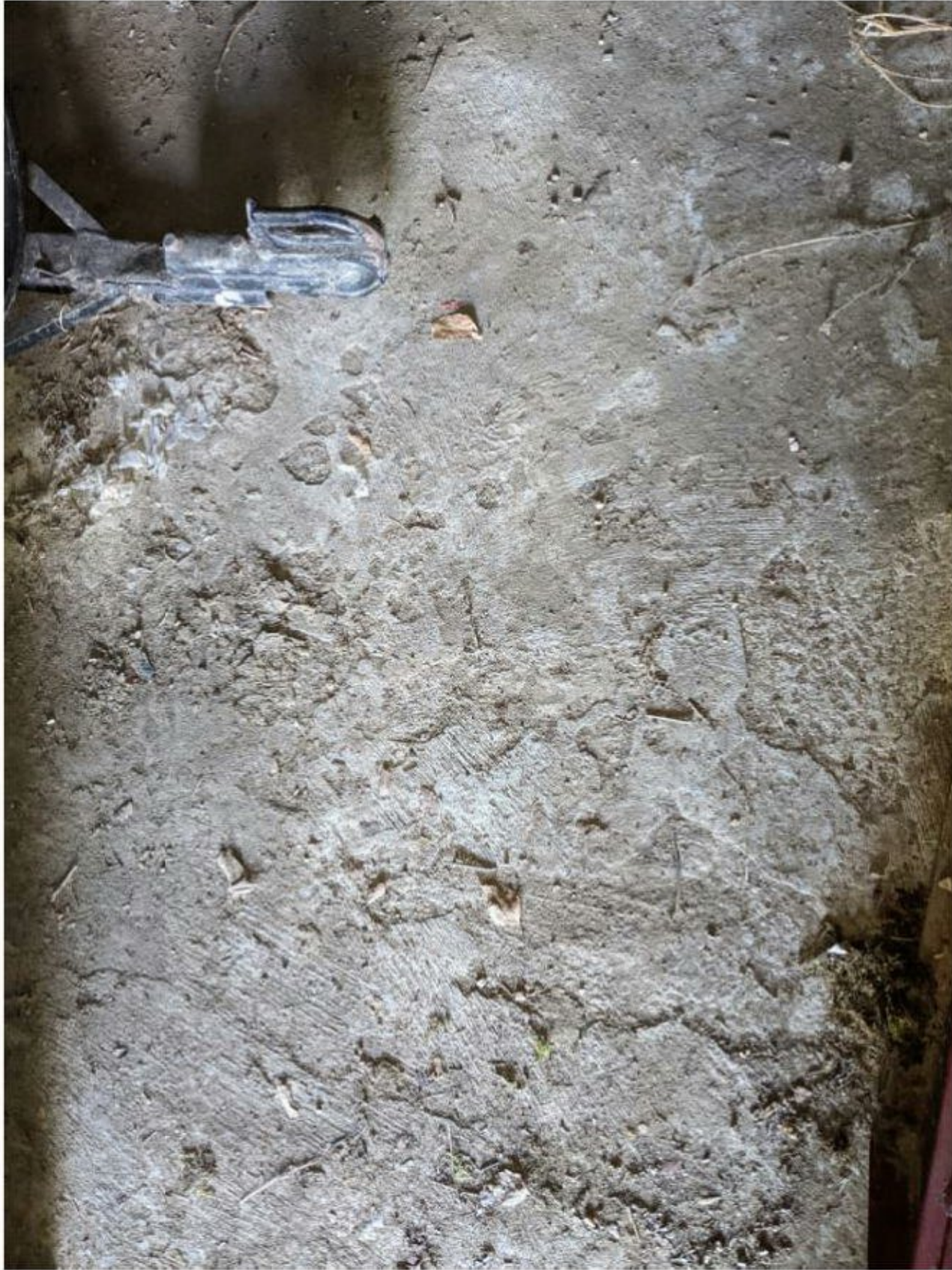
Figure 30 Concrete floor slab inside The Barn
