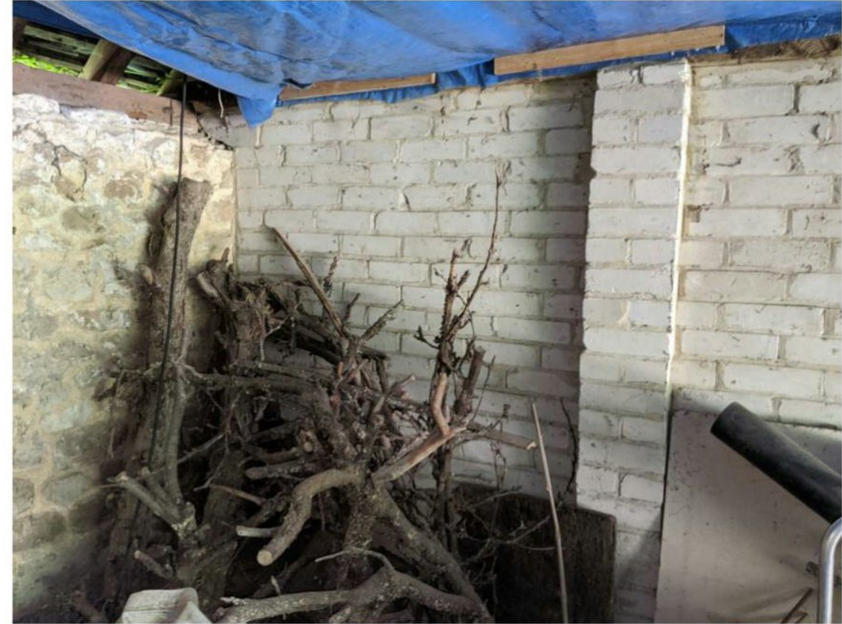
Figure 23: Later white brick partition, which subdivides the barn.
