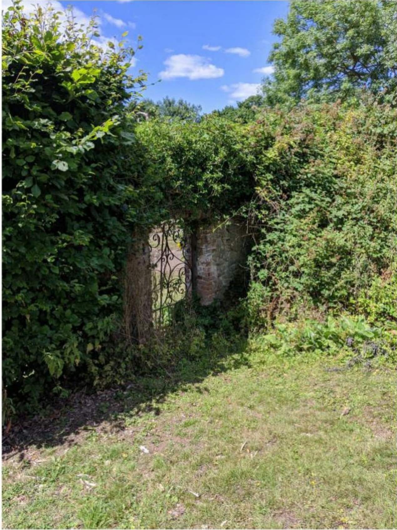
Figure 31: The grade II listed garden walls.
