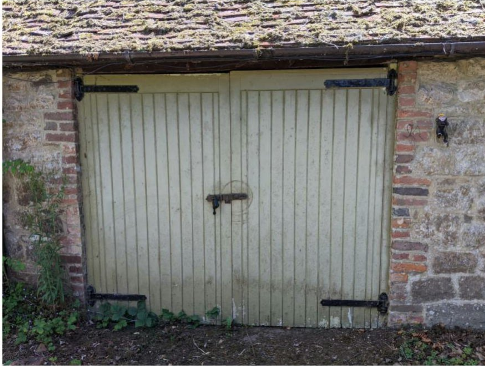
Figure 20: The central doorway to the barn. North elevation.
