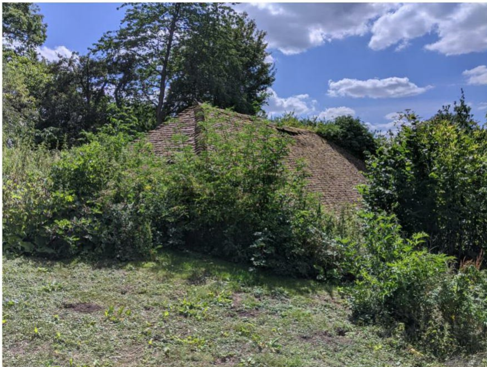
Figure 18: East elevation of the barn. The land slopes up and conceals a large section of the elevation.
