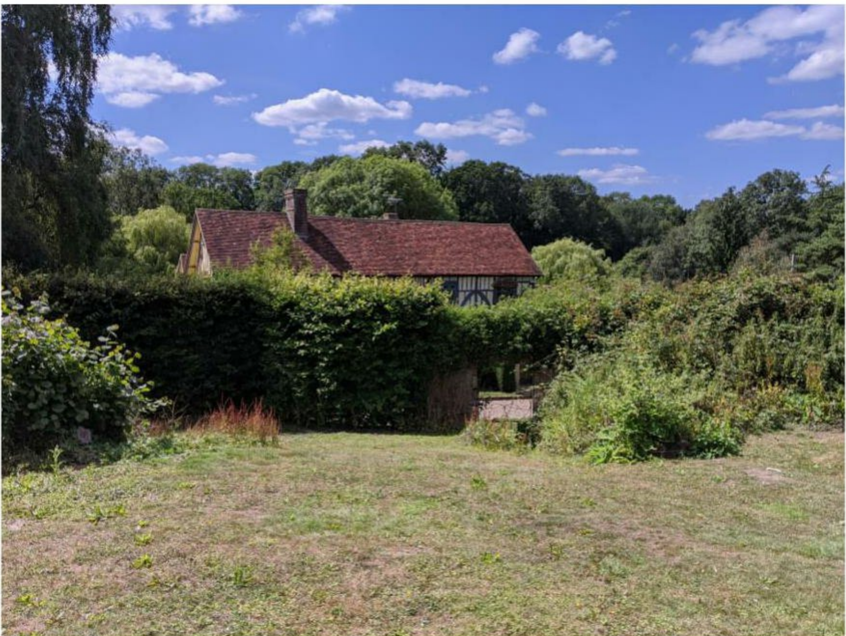
Figure 19: View towards Dryhill Farmhouse from the barn's north elevation.
