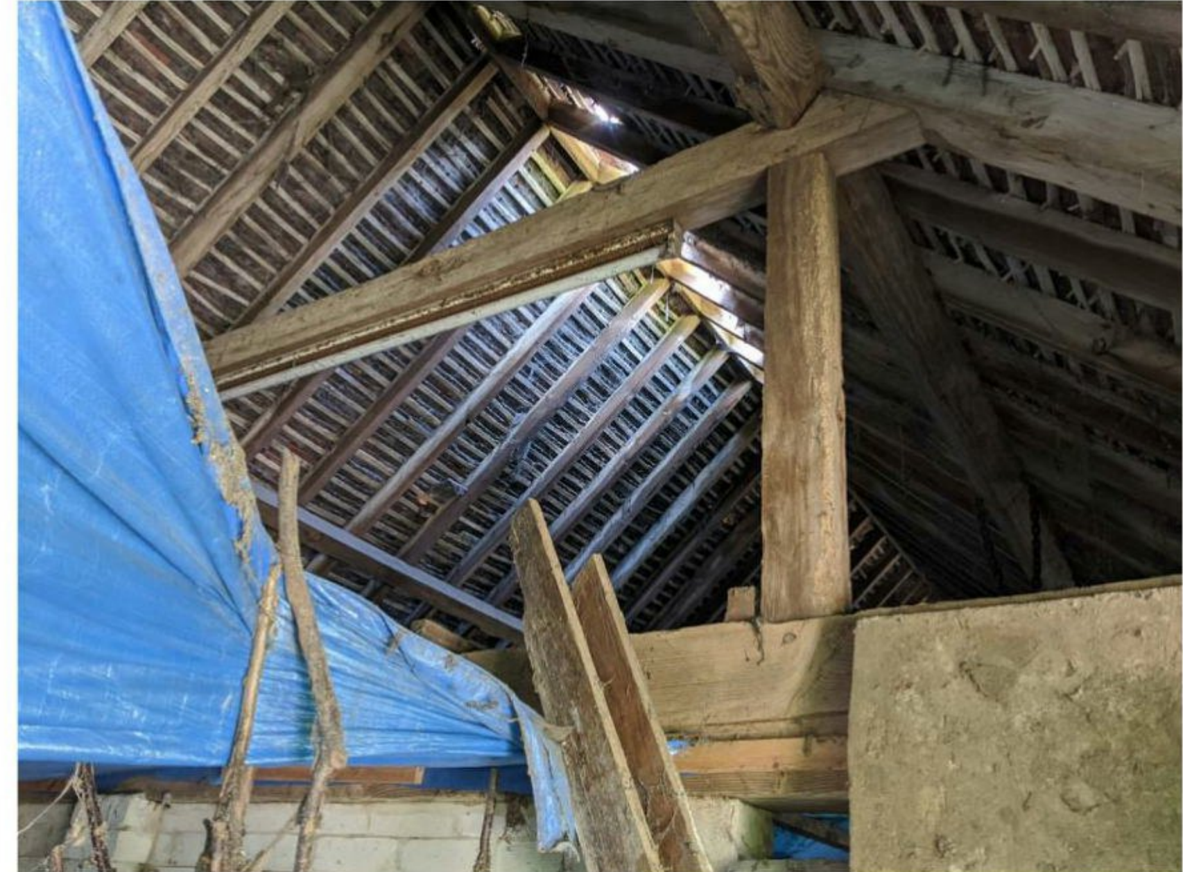
Figure 27: One of the two open queen post trusses.
