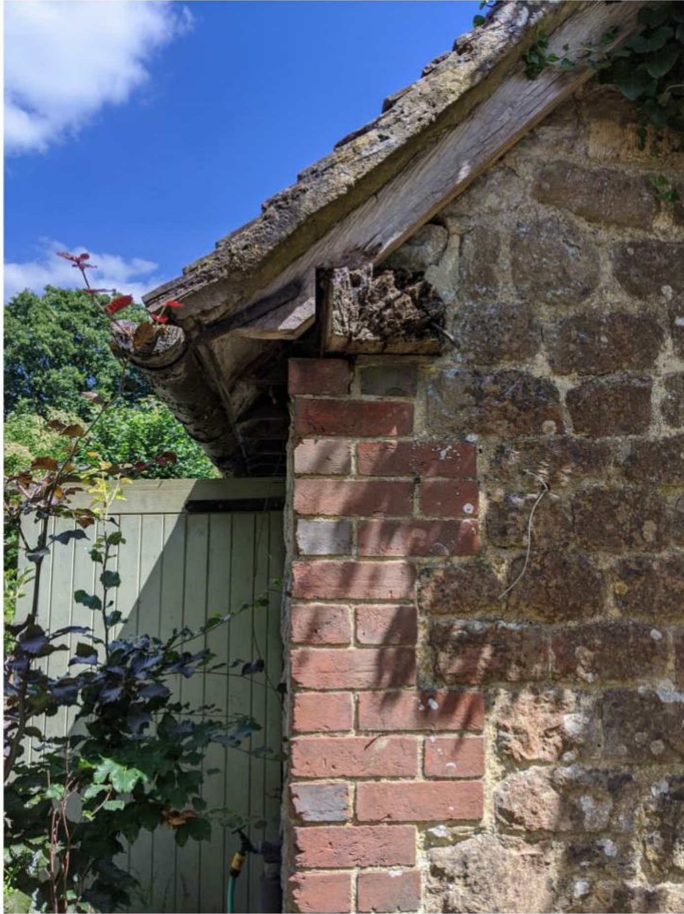
Figure 28: East/north corner showing a different type of stone and the red brick quoins.
