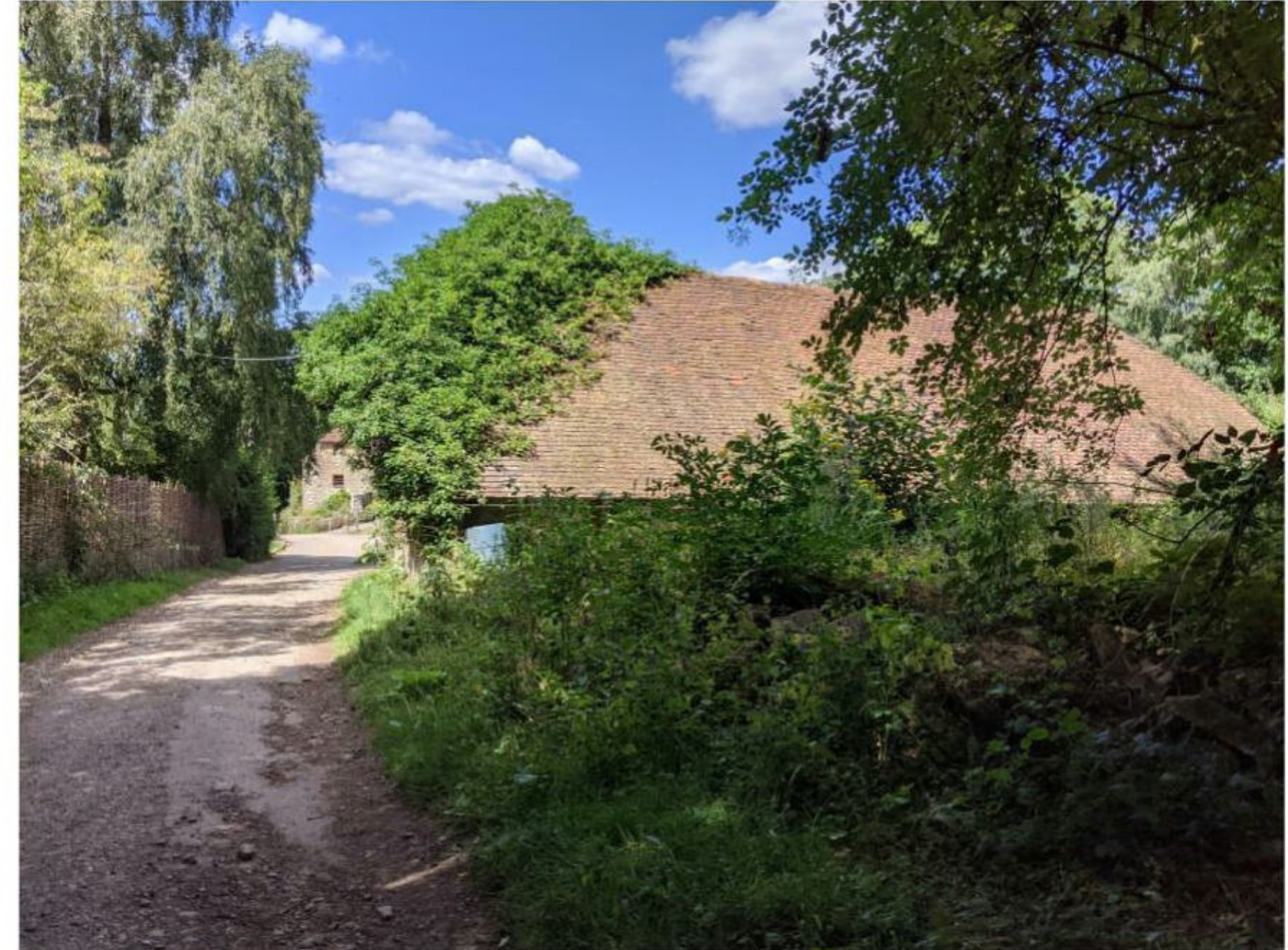
Figure 21: Similar to Figure 17, view looking north from the west elevation of the barn. Central to the view is the grade II listed outhouse.
