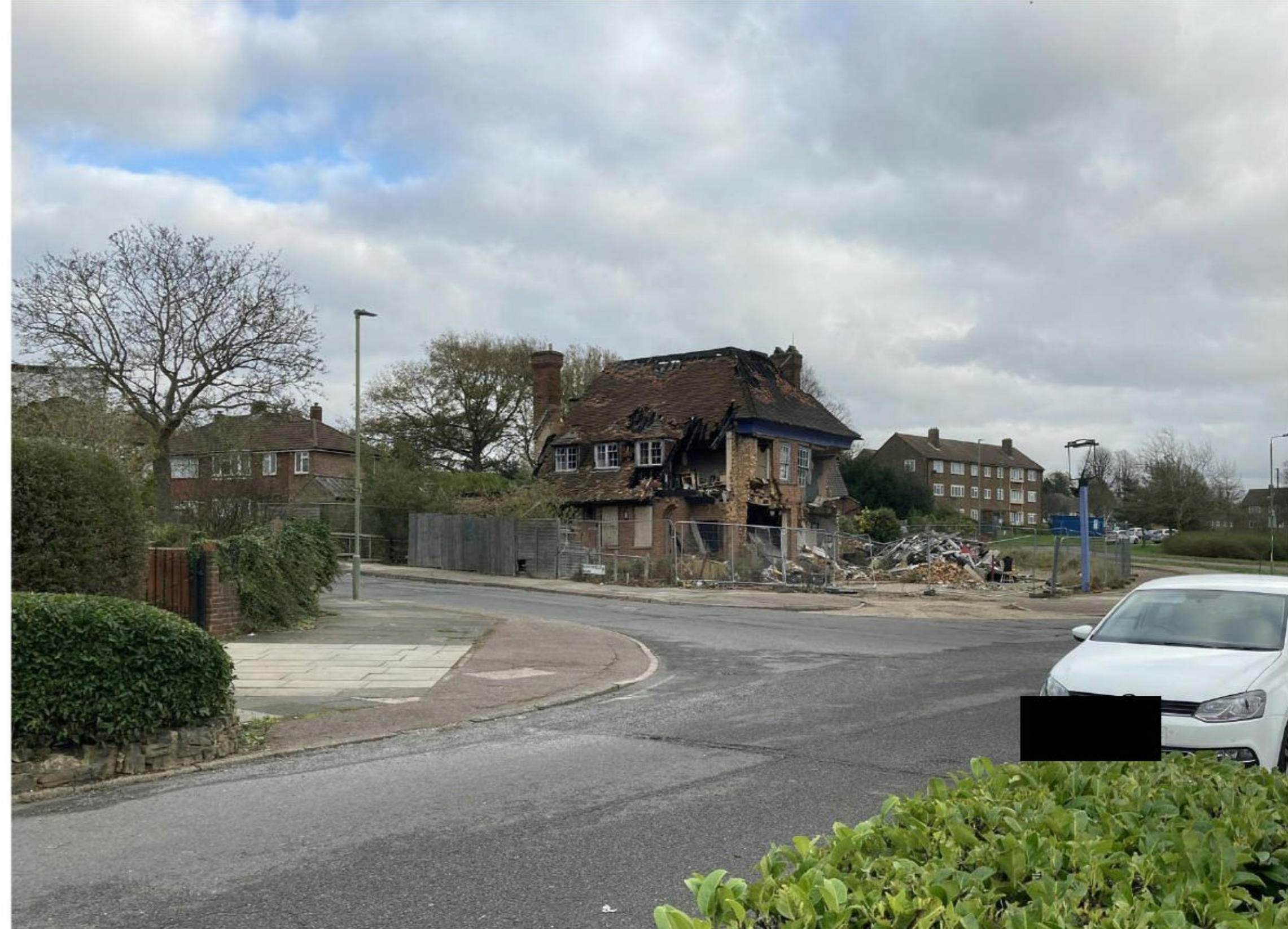
150 Mt Pleasant, existing condition
