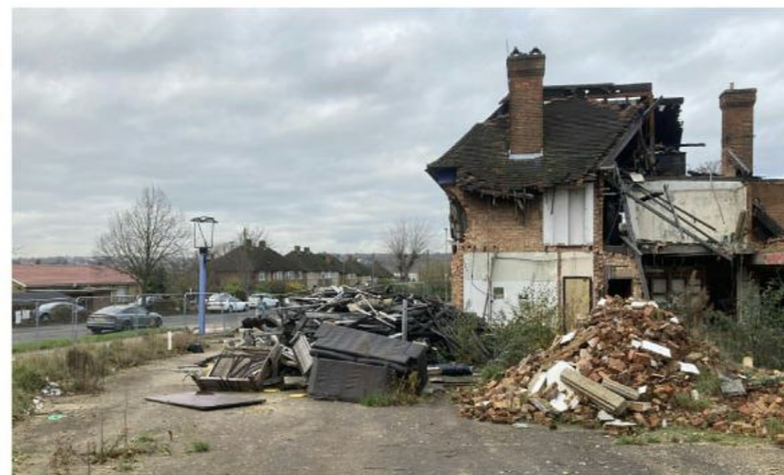
Current state of building
