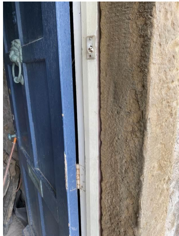
Existing photographs of door
