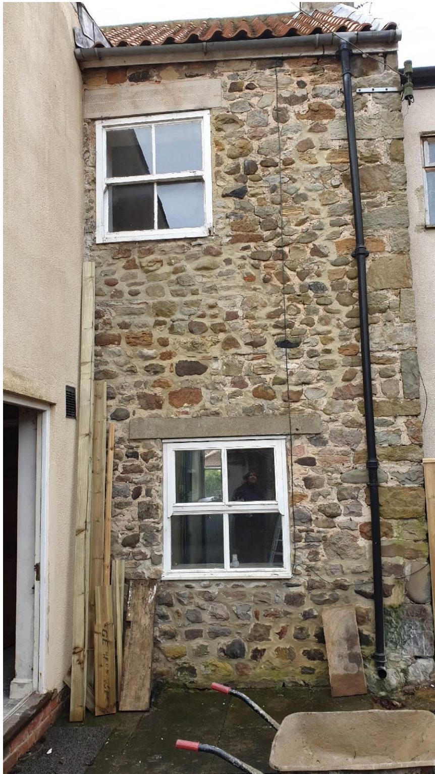
Example of windows to the rear of the property
