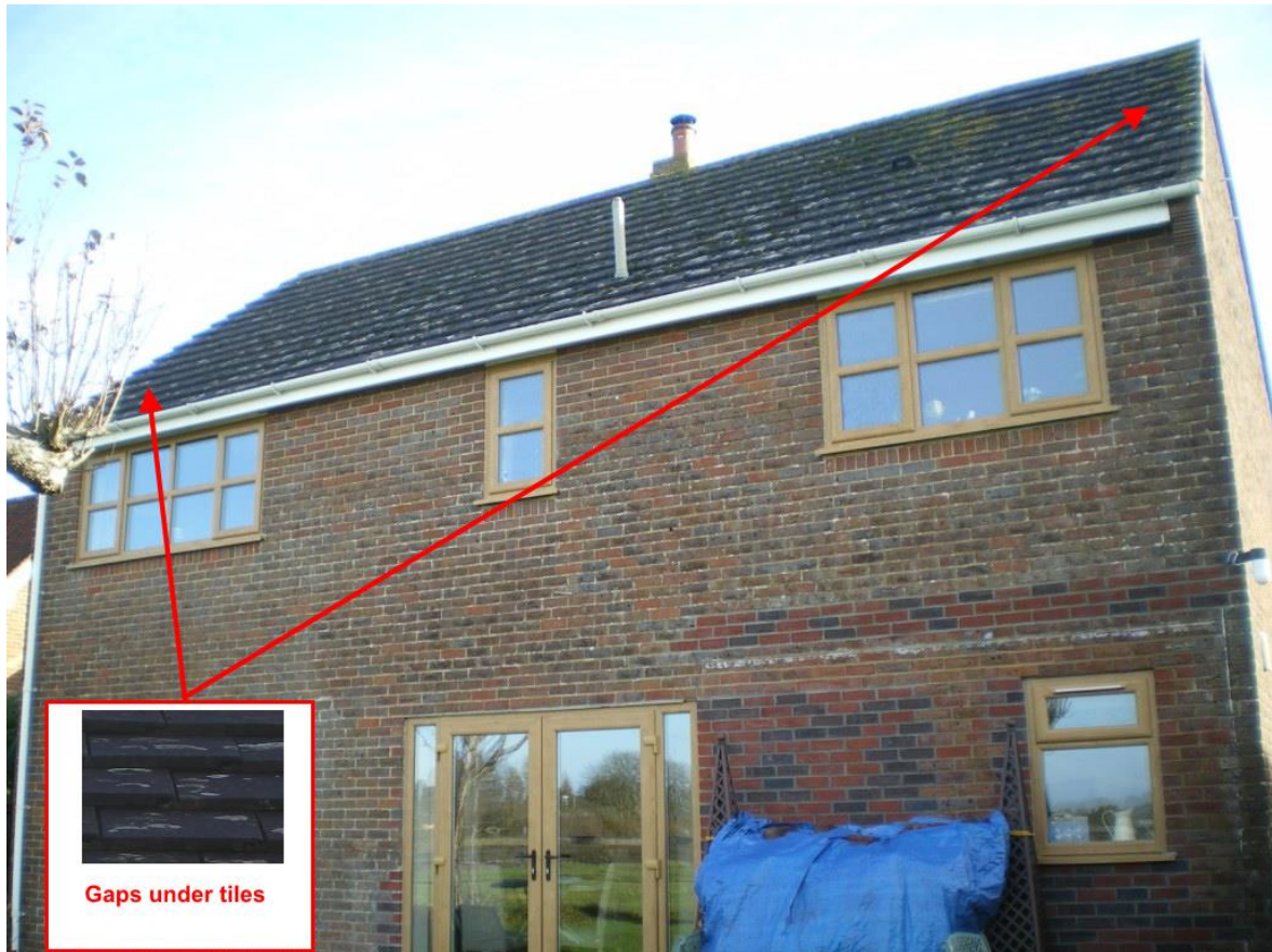
Image 4.3.1. Location of potential bat access points and potential external roost locations on the north-west elevation of the building.
