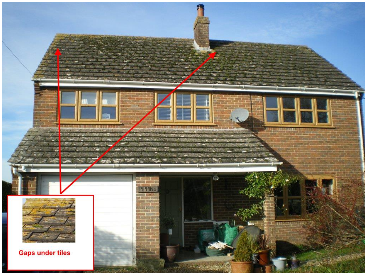
Image 4.3.1. Location of potential bat access points and potential external roost locations on the south-east elevation of the building.
