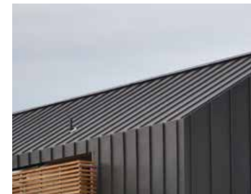
3. Black zinc roof with seam
