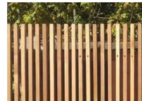
4. Timber detailing and fencing
