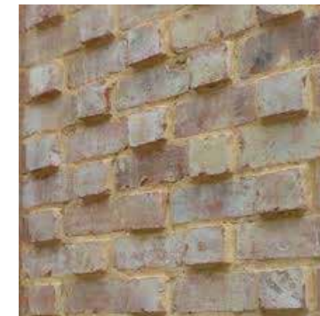
2. Brickwork detailing at entrance
