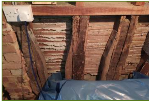
Early timber in the staircase to the cellar.
