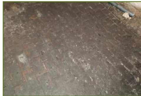
Cellar's original floor.
