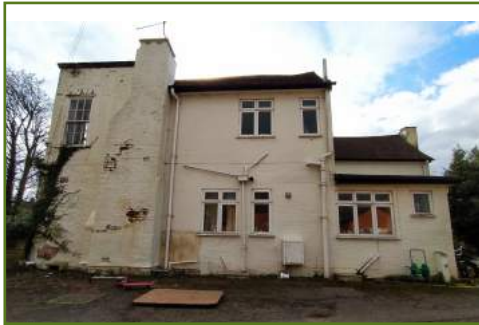
North-east elevation of The Old Vicarage.
