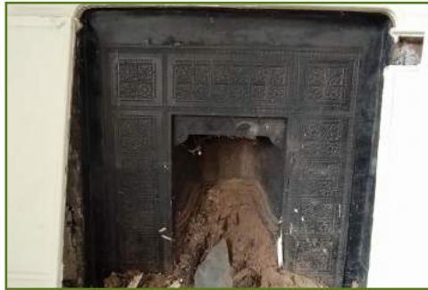
Concealed Victorian iron cast fireplace.
