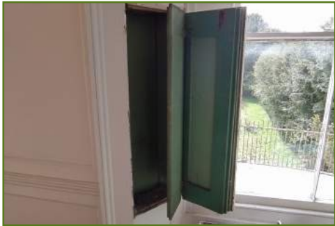
19 th century window shutters.
