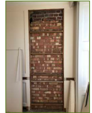
Modern brickwork blocking original doorway.
