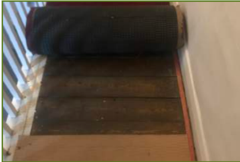
Modern joists and floorboards forming landing to bedroom over drawing room.
