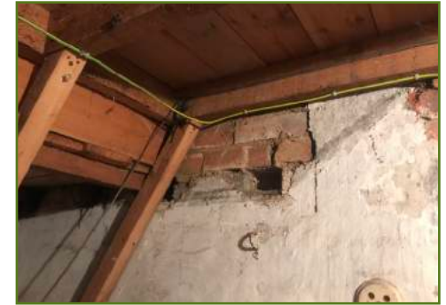
Modern brickwork upwards from height of original quarter landing. Evidence also of staircase being full width of stairwell incorporating what is now the cupboard.
