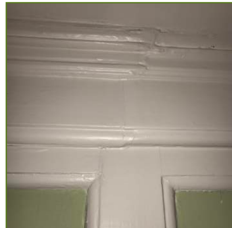
Panel join lines.
