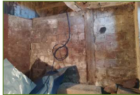
Upper landing of the cellar's staircase
