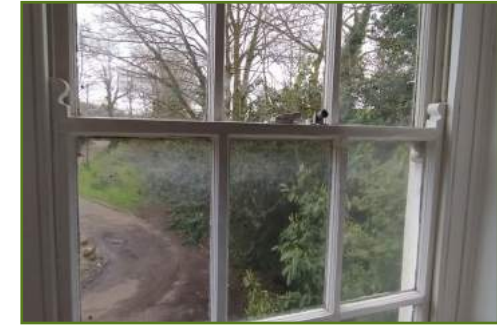
Detail of sash window frame.
