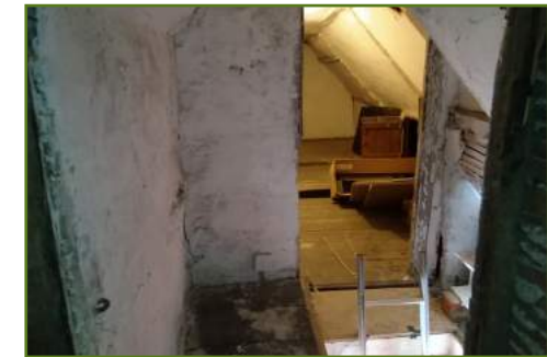
Former stairwell in the loft.
