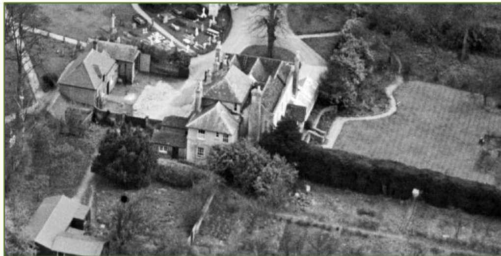
Aerial view of The Old Vicarage from the north-west, 1937.
