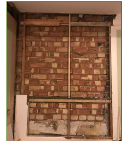
Modern brickwork found behind panelling.
