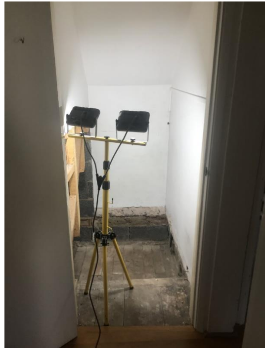
Photo of under stairs showing original brick floor
