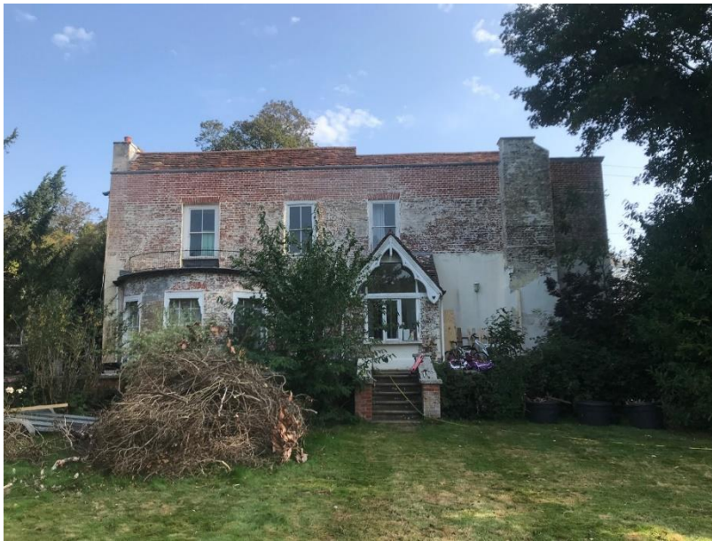
SW Elevation from the garden with some of the paint removed
