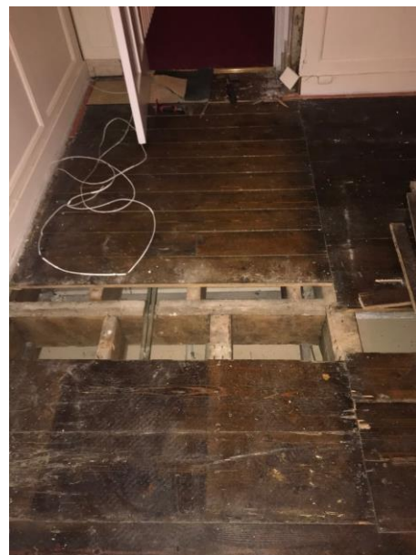
Photos from position 5 showing join line of flooring – then opened up showing trimmer and landing
