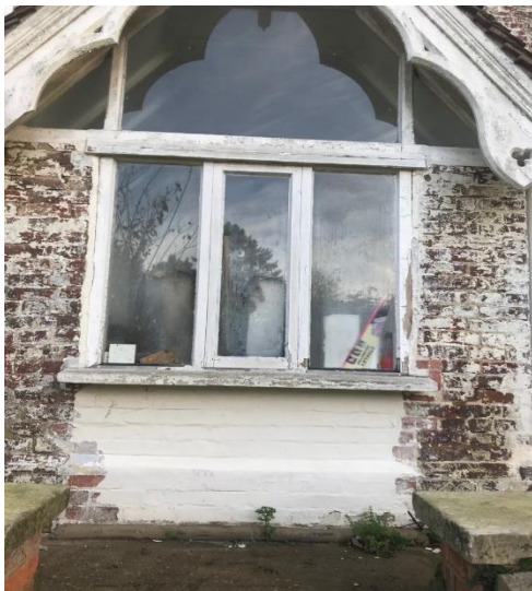
Garden face of porch showing modern bricked up section and original step
