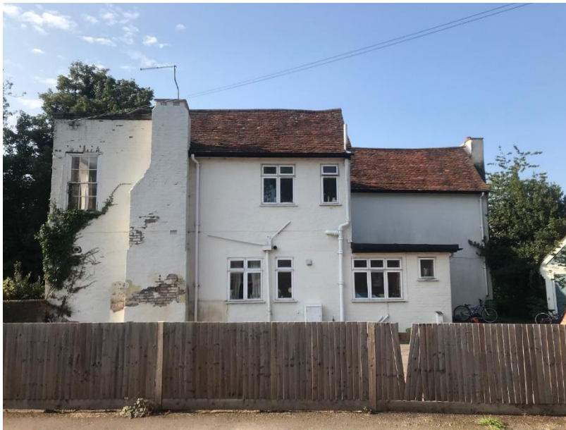
View of the NE Elevation from the Old Stables
