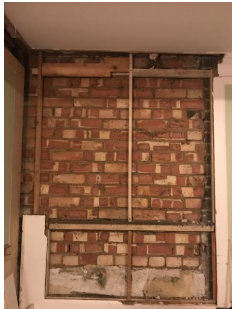
Photos from position 3 showing panel join lines and after carefully opening up panelling
