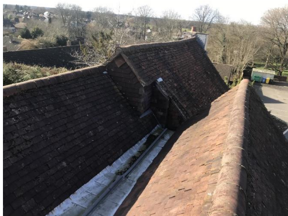
Roof as existing
