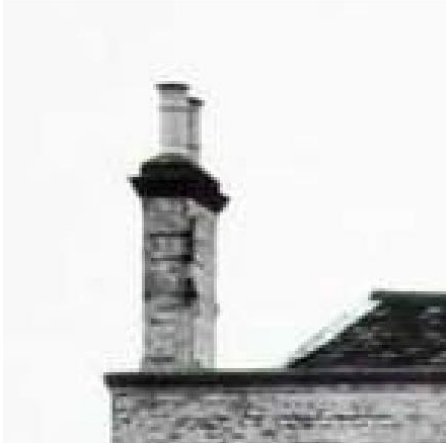
Photograph of original chimneys (see HBA)
