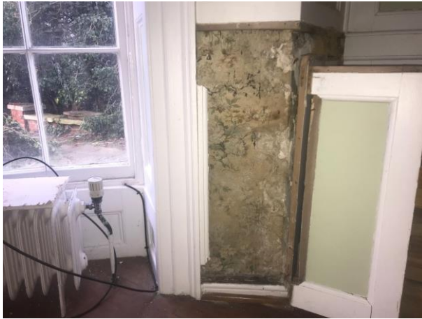
Photos from position 4 showing wall paper full height behind panelling
