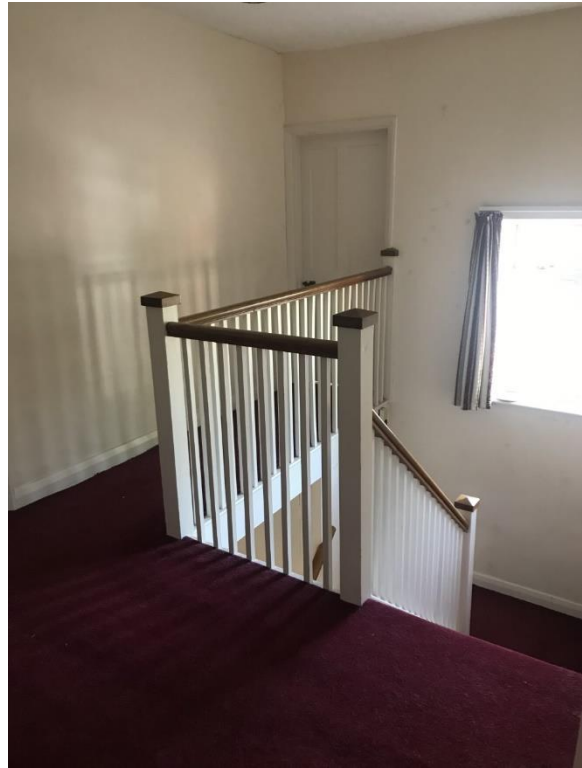
Stairway viewed from upper landing
