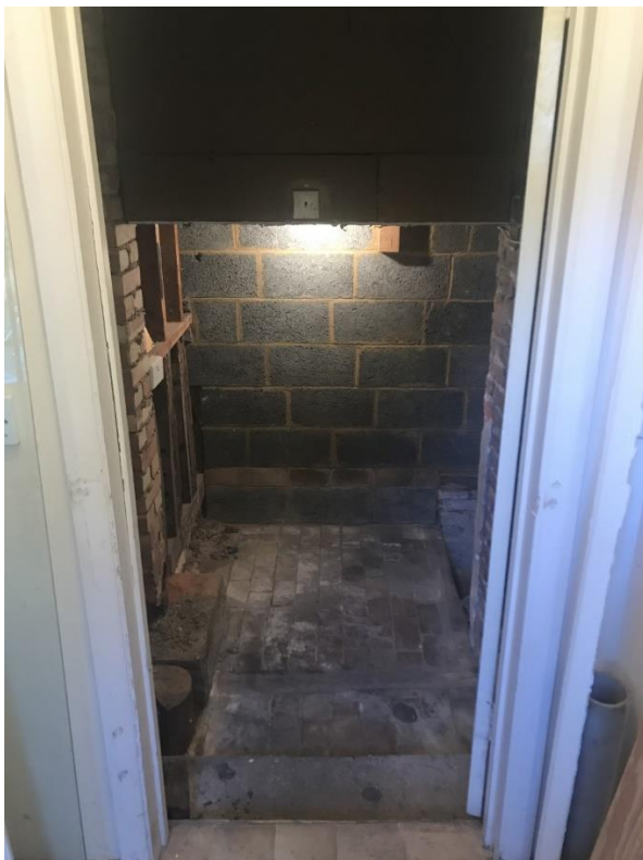
Photo of entrance to basement stairs showing original brick floor
