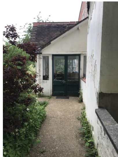
Existing porch with old double doors
