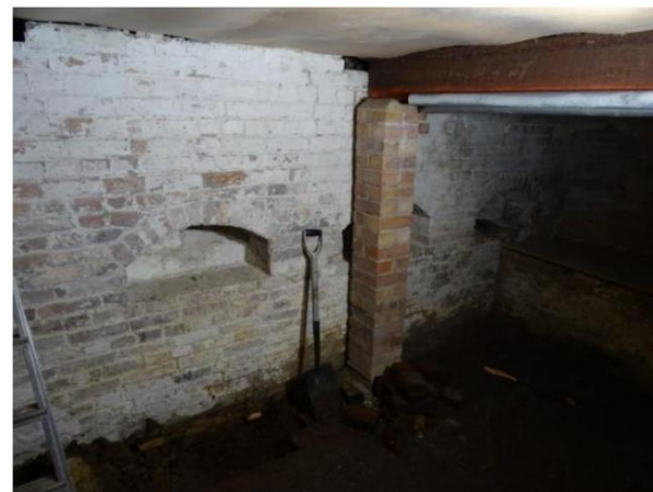
Basement under dining room with modern pillar
