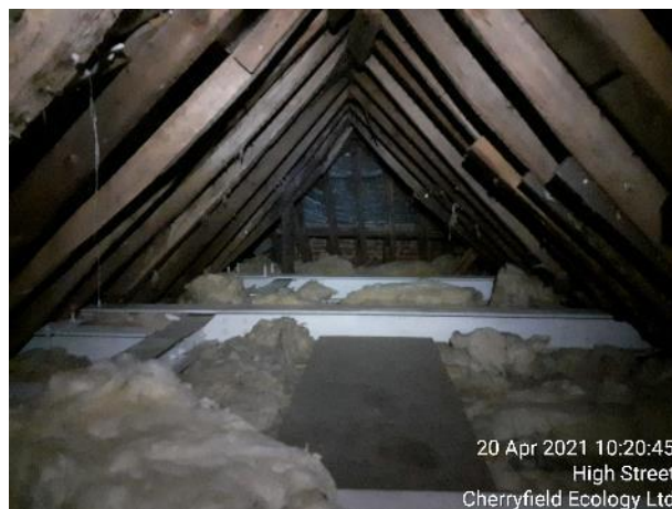
Figure 8: Example of B1's loft space.
