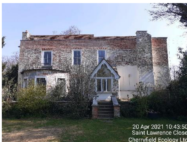
Figure 2: Front elevation of B1.
