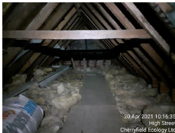
Figure 7: Example of B1's loft space.
