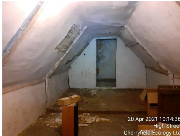
Figure 6: Example of B1's loft space.
