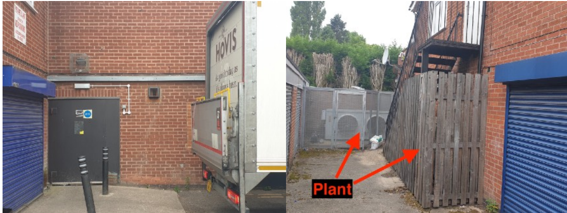
Figures 3 & 4 : Rear delivery door and plant area
