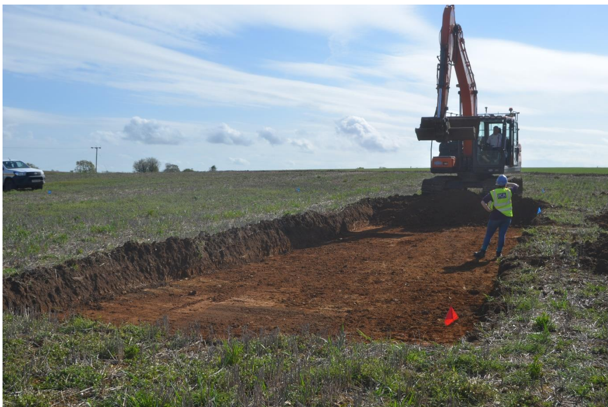
Plate 1: Working shot of site, view east.
