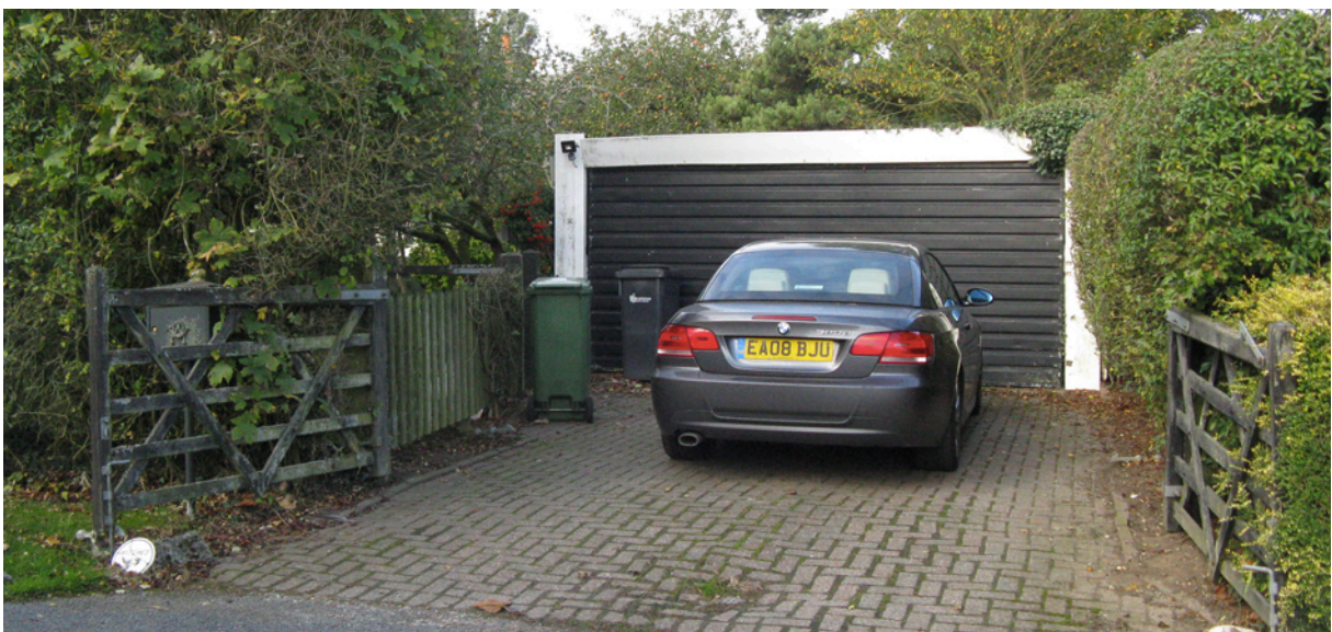
Figure 3 | The off-street parking and existing double garage
