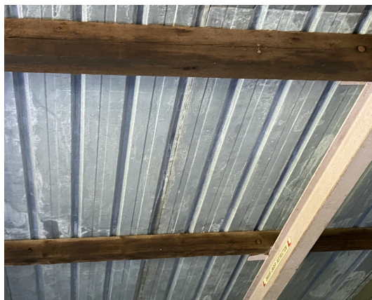
PHOTO 6 - Neatly installed, good condition roof sheets over garage
