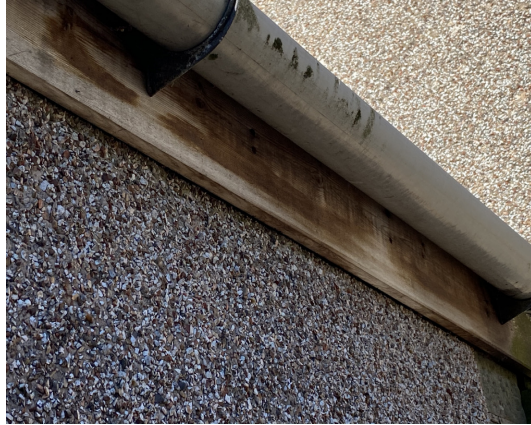
PHOTO 7 - Garage fascias soffit detail - no gaps
