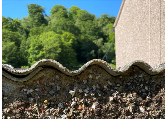
PHOTO 4 - Render beneath corrugated sheet
