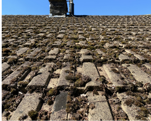
PHOTO 1 - Neatly butted tiles
