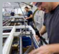
FABRICATE NEW WINDOWS
