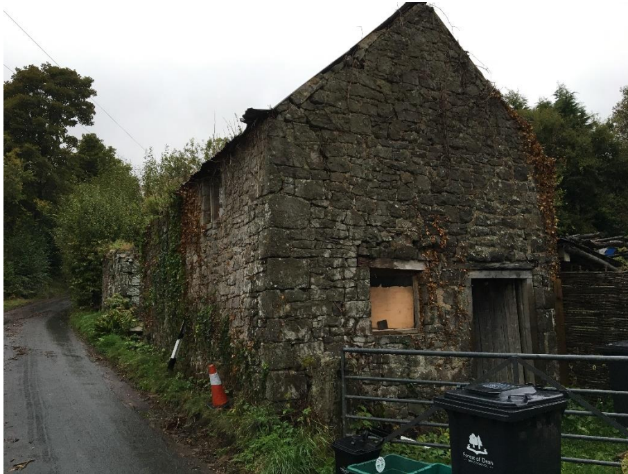
Figure 2- Barn south elevation
