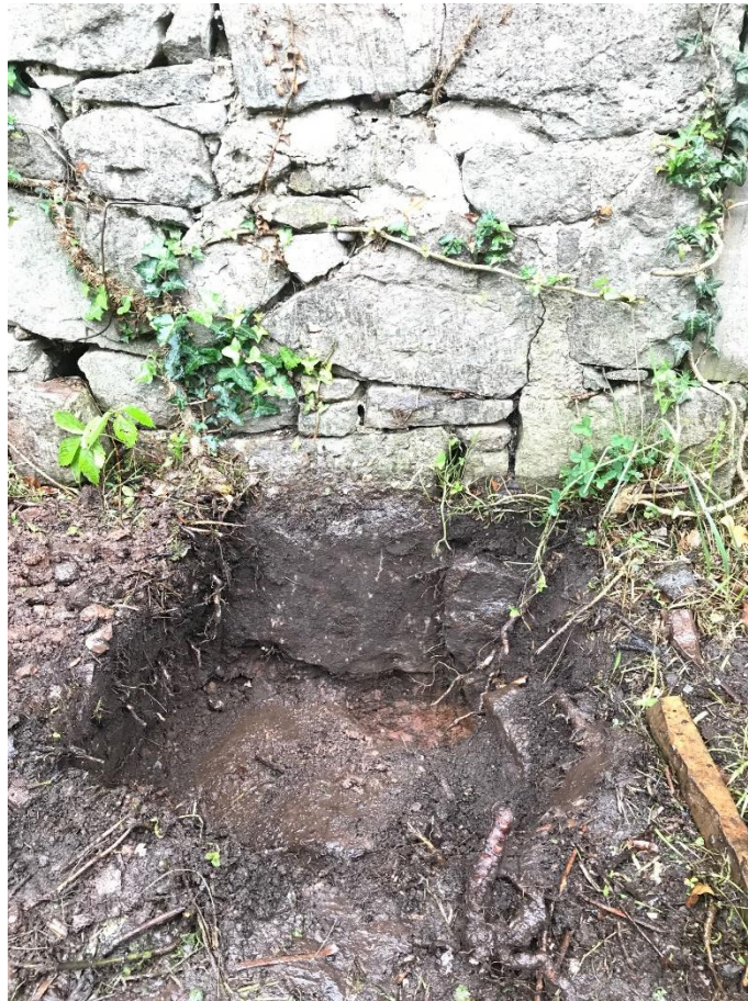
Figure 5- Additional trial pit showing large stone footings
