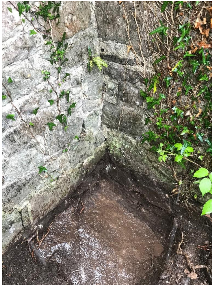
Figure 4- Trial Pit showing large stone footings
