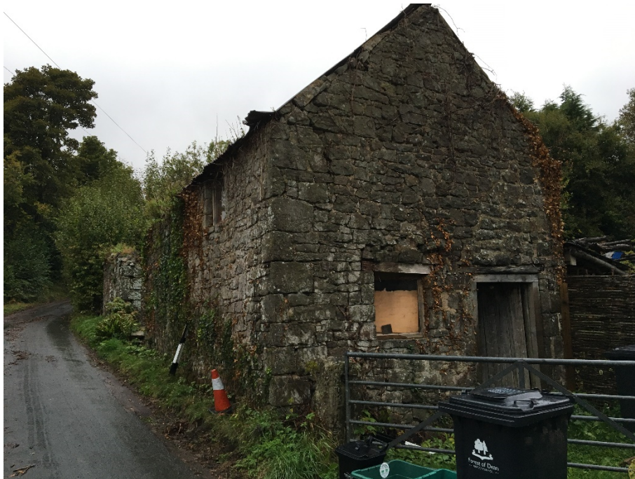
Figure 1; Front elevation of the barn.
