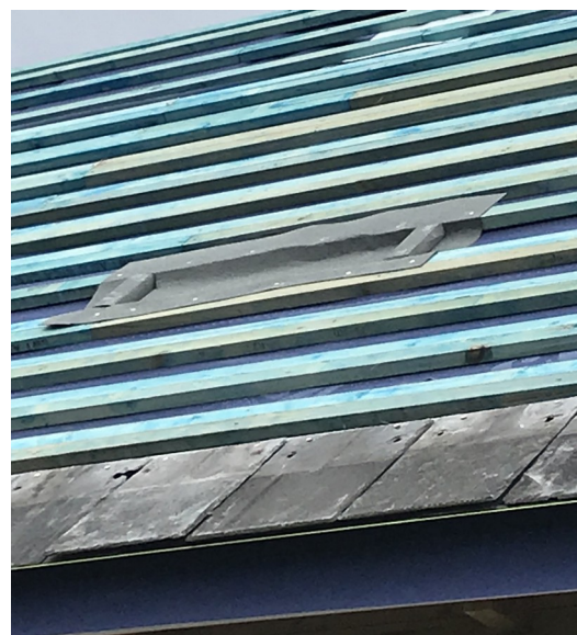
Ref: Bat 2 East facing 'Just Lead bat access slate' with 1F bitumen felt enclosure
