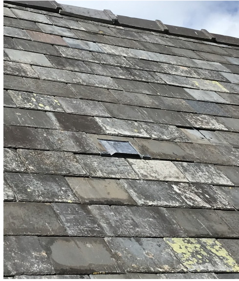
Ref: Bat 2 East facing 'Just Lead bat access slate' with 1F bitumen felt enclosure
