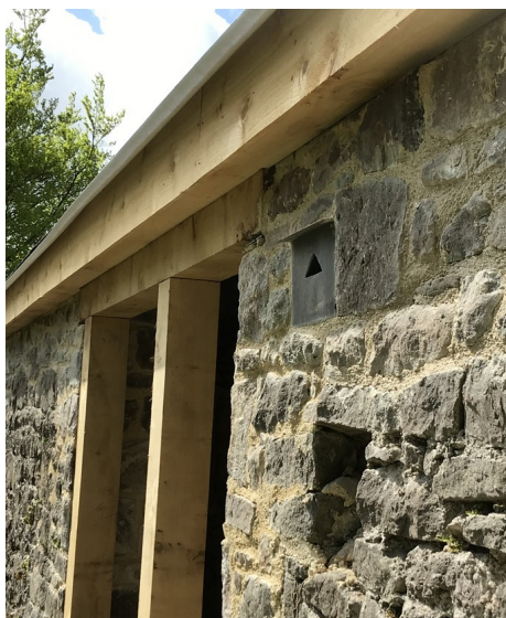
Ref: Bird 3 East facing NHBS WoodStone Build-in Open Nest Box faced with slate facing Product code: 5051054183688 Installed March 2021
