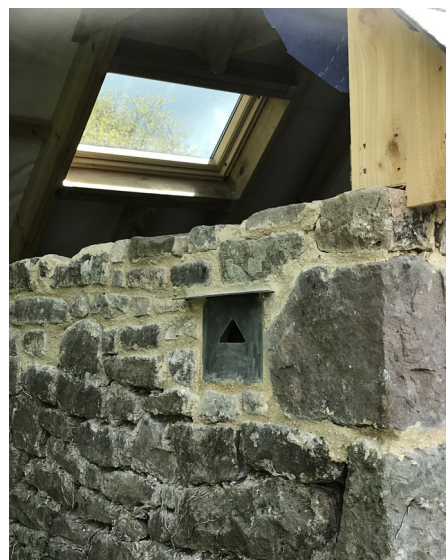
Ref: Bird 4 North facing NHBS WoodStone Build-in Open Nest Box faced with slate facing Product code: 5051054183688 Installed March 2021
