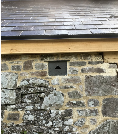
Ref: Bird 1 West facing NHBS WoodStone Build-in Open Nest Box faced with slate facing Product ode: 5051054183688 Installed March 2021
