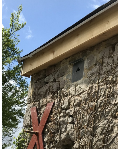
Ref: Bird 2 East facing NHBS WoodStone Build-in Open Nest Box faced with slate facing Product code: 5051054183688 Installed March 2021
