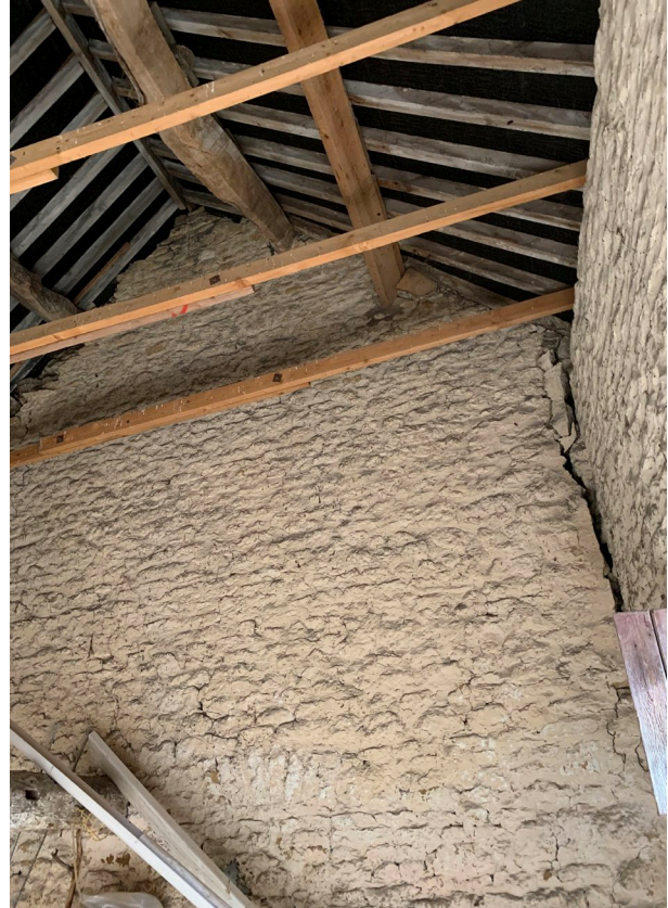
Figure 8: View of the junction between the Bull House and Wisteria Cottage
