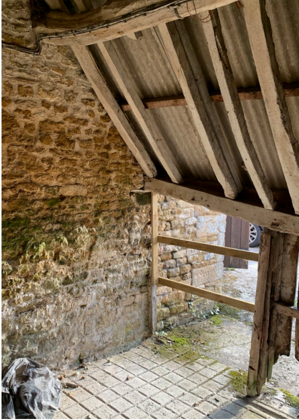
Figure 4: View of the low eaves condition of the single
