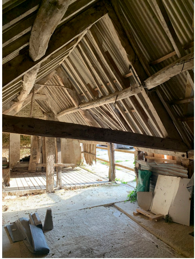
Figure 5: View of the single storey barn looking towards the Bull House
