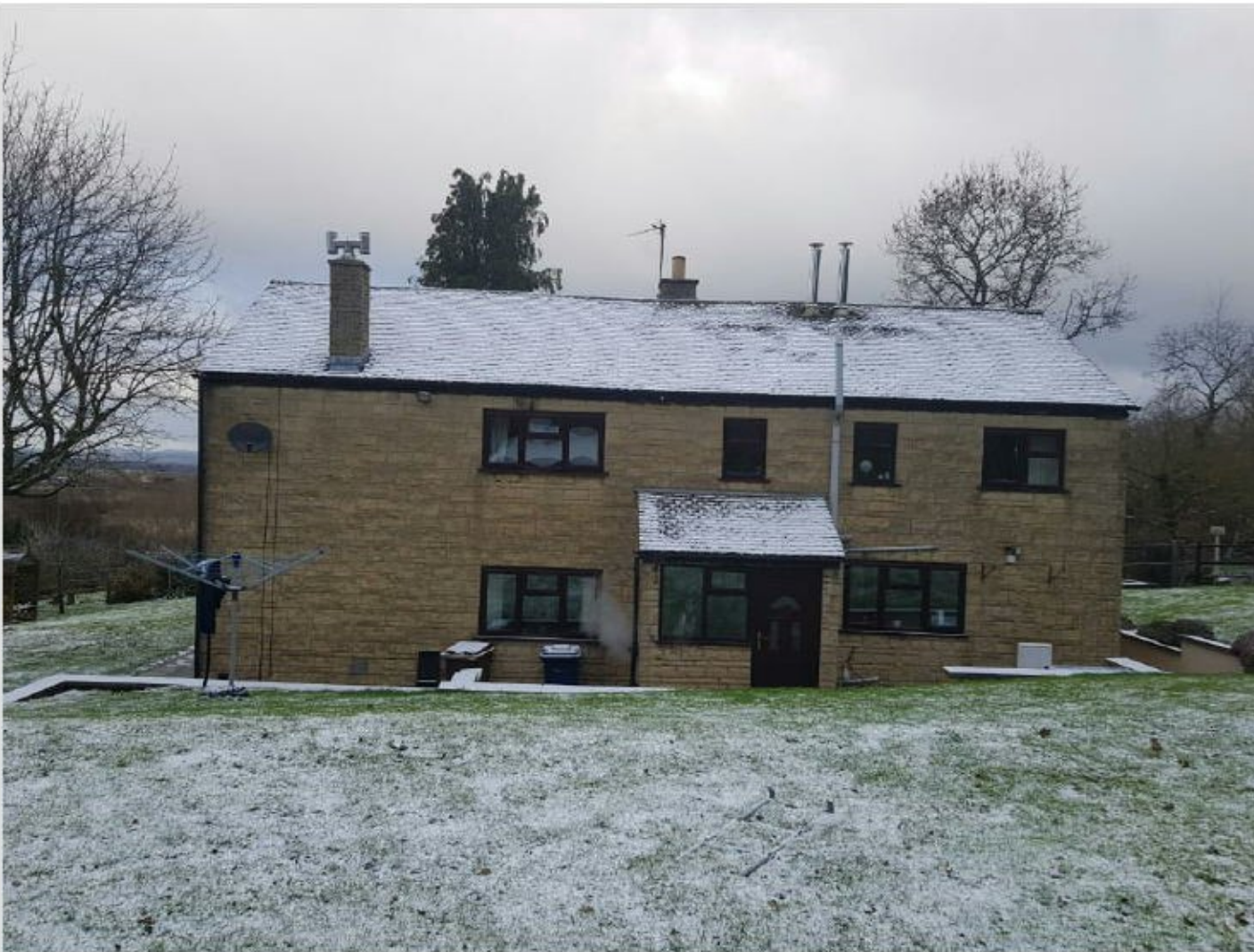
Figure 3 showing the dwelling's existing southern elevation
