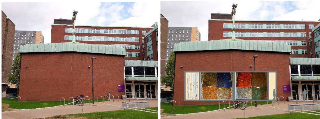
Photograph showing the existing elevation and roof-top Michael Piper Sculpture, Schuster Building Lecture Theatre wall with mosaics superimposed.
