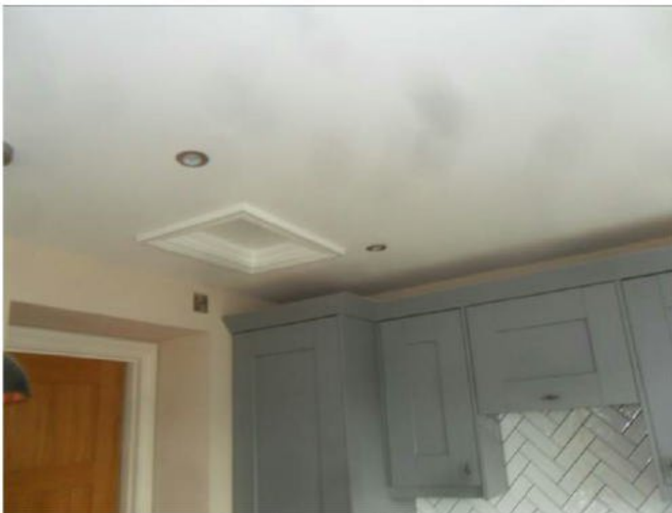
Access hatch out of kitchen
