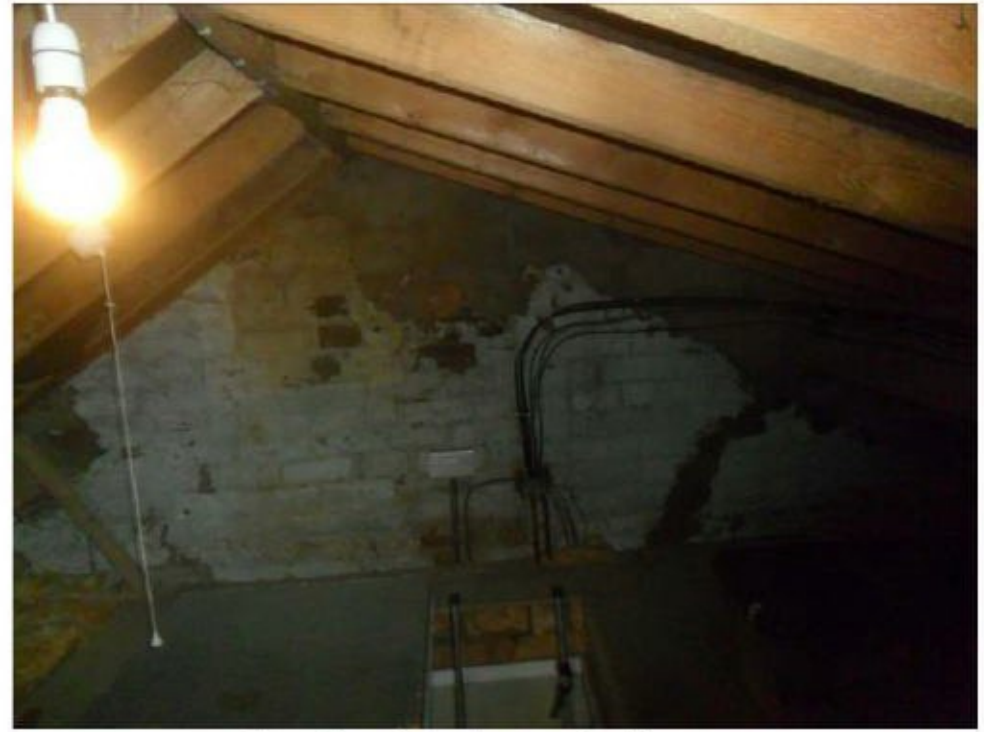
Roof void above bedroom
