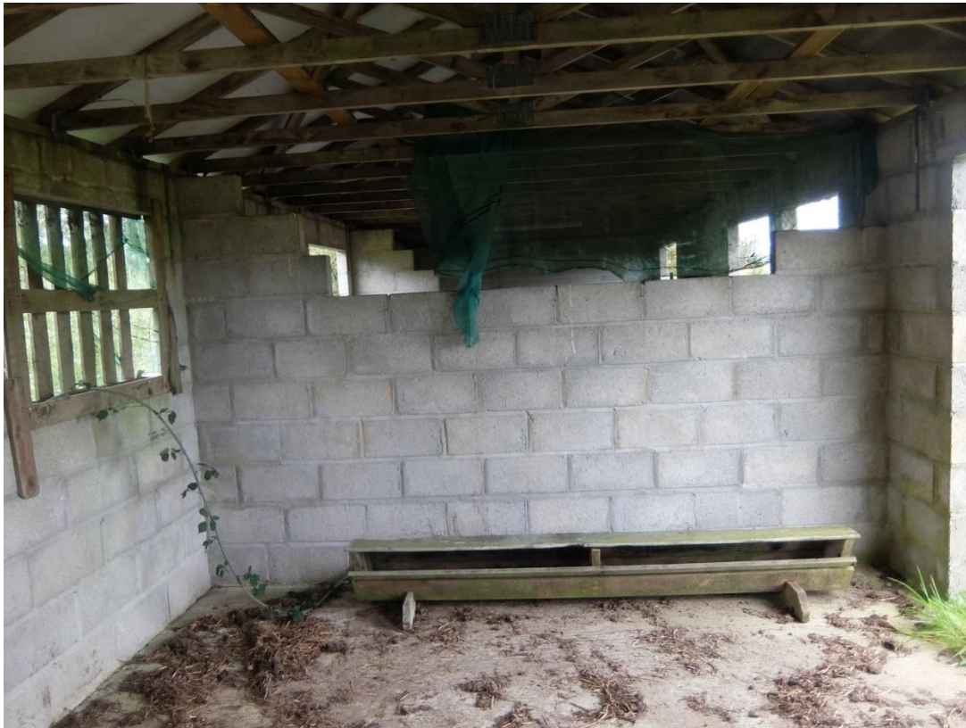
Internal view within Bay 9 looking towards front
