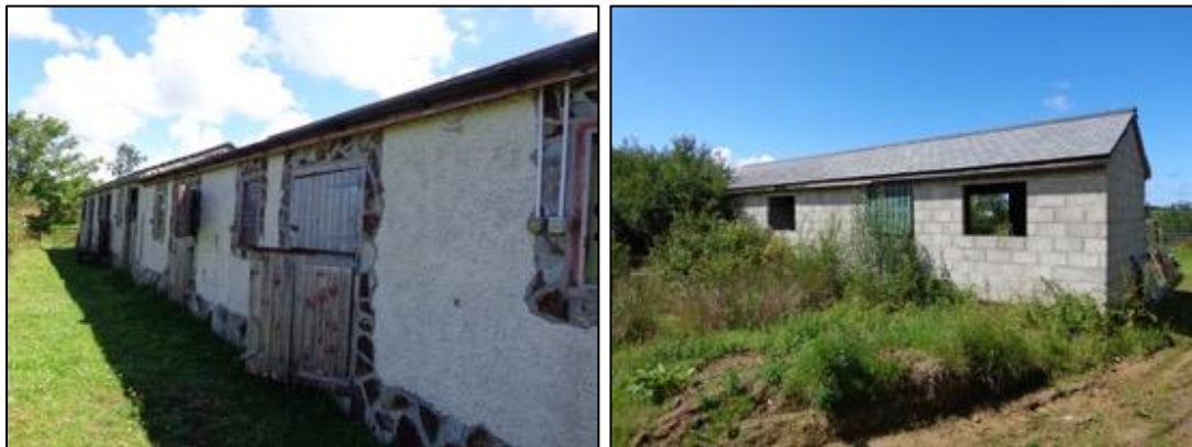
Figures 1 & 2. Barn viewed from the south-west [left] & north-east [right]
