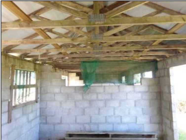
Figure 3. Interior view of barn
