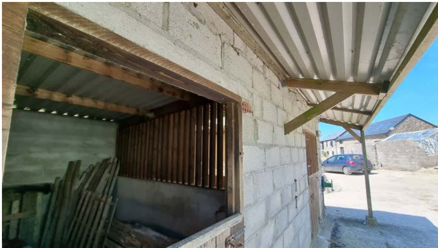
Photograph 9 – Concrete lintel to stable opening.
