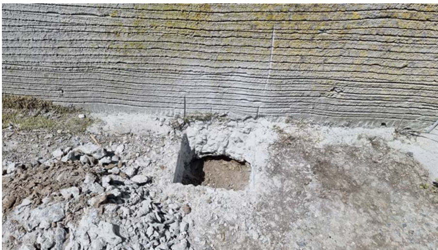
Photograph 5 – Trial pit excavated to eastern end of building
