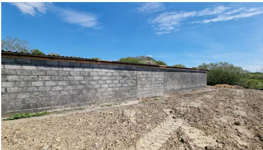
Photograph 4 – Masonry infill panel to rear flank wall
