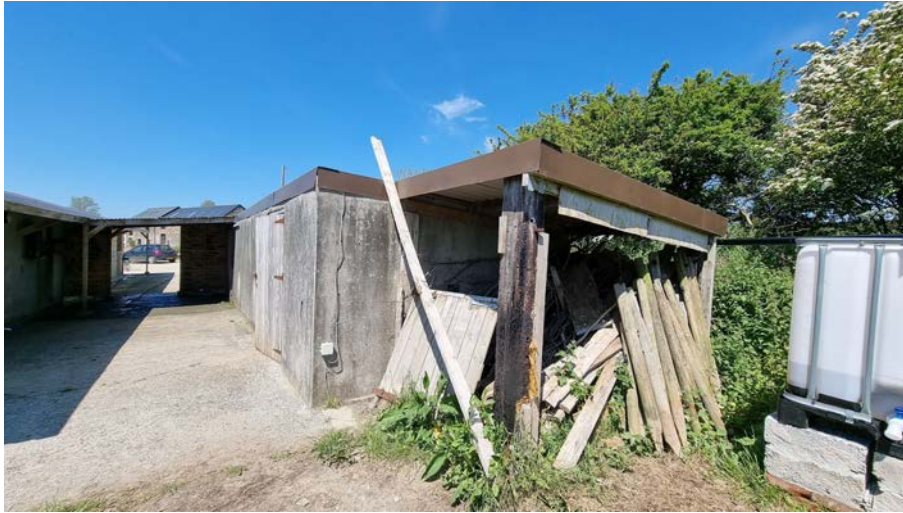
Photograph 10 – Timber frame addition to eastern end
