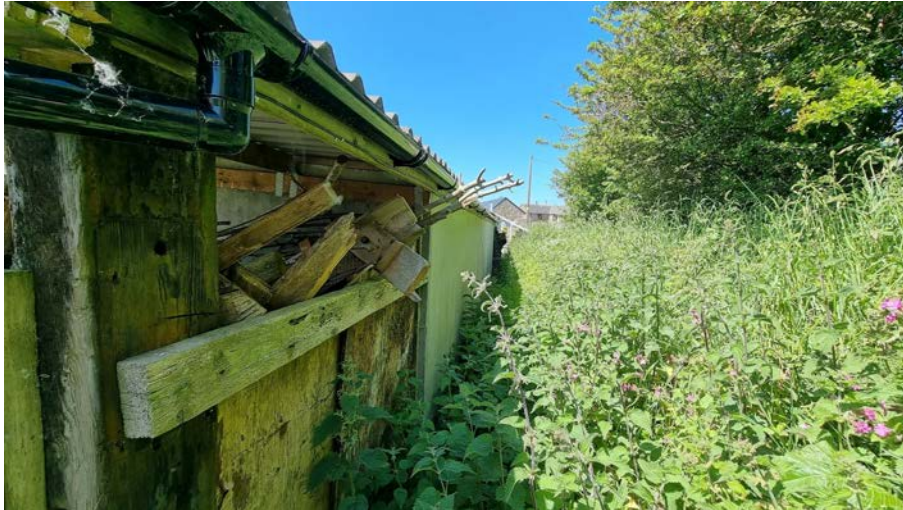
Photograph 5 – Foliage build up to flank wall
