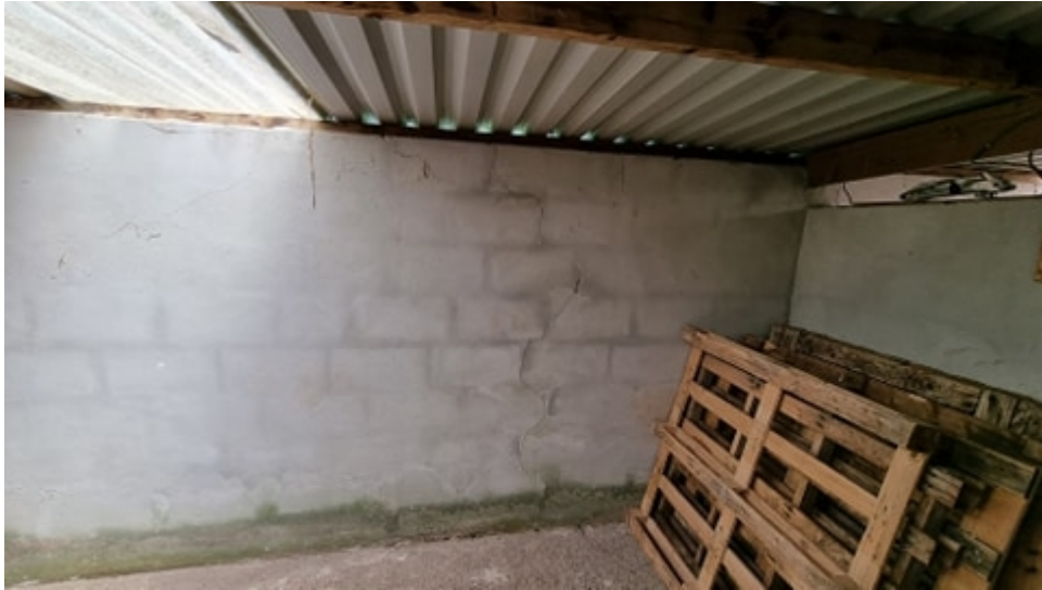
Photograph 3 – Cracking to flank wall of shorter barn
