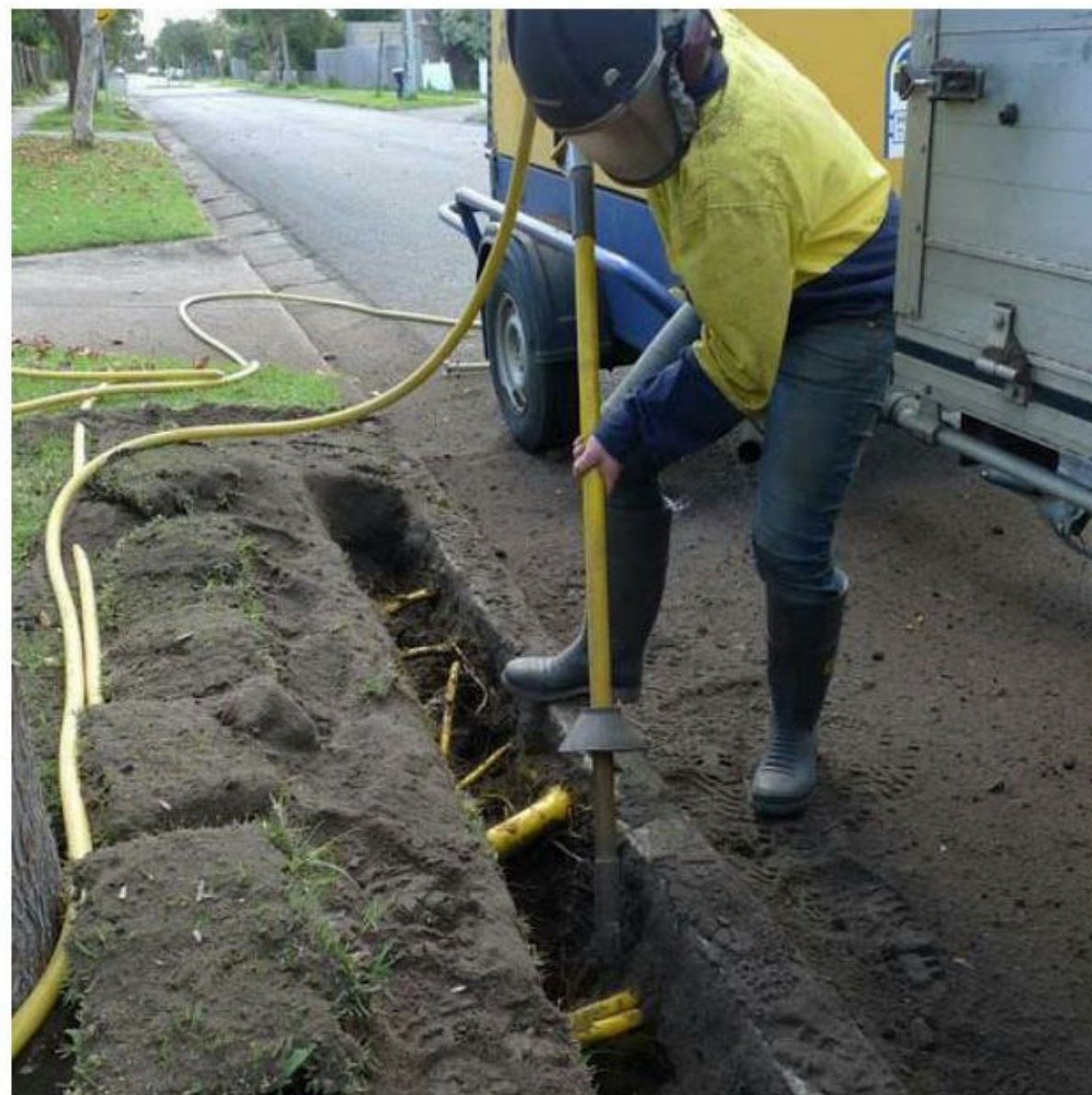
Image 6 -Air Spade excavation (Sandy/Loamy soils only. Vacuum excavation of loosened soil in recommended)
