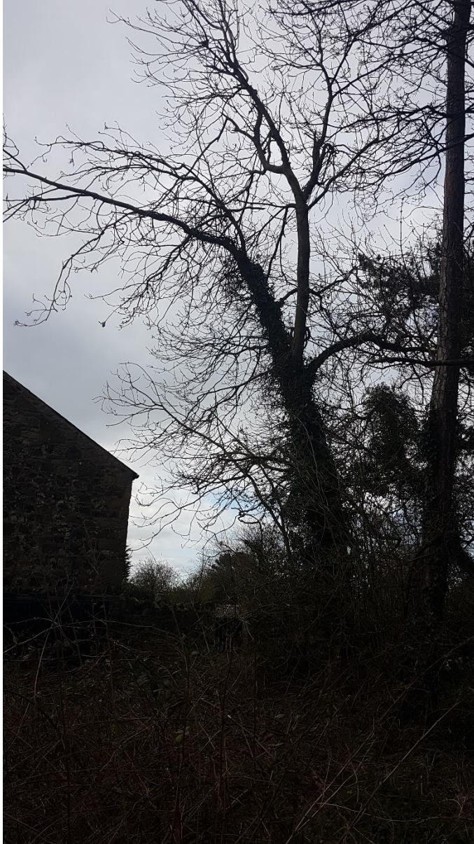
T1 Ash showing signs of dieback and a lean towards a neighbours house.
