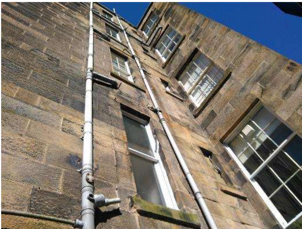
4. General photo of existing WC window
