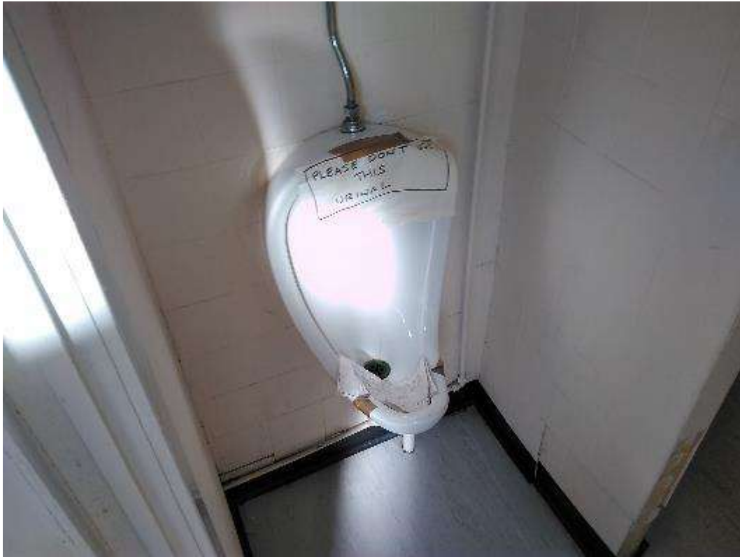
7. Urinal – to be removed
