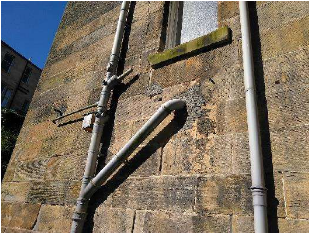
3. External connection to SVP – to be retained.
