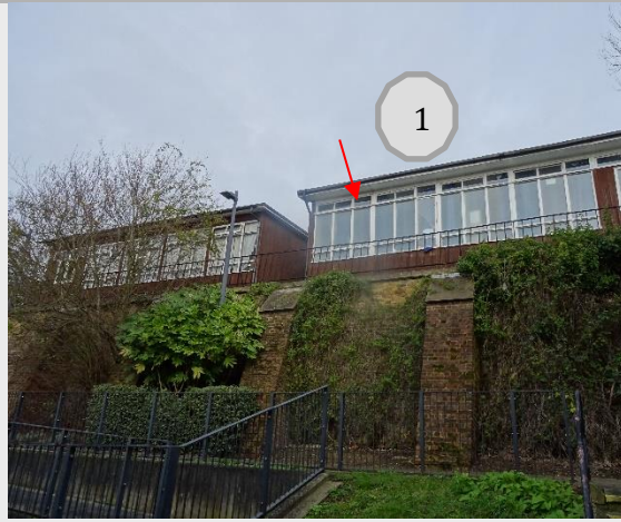
Photo 9. South facing elevation
