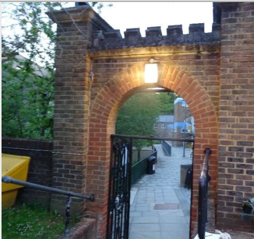
Photograph 1. Nearby lights reflecting onto north elevation of buildings
