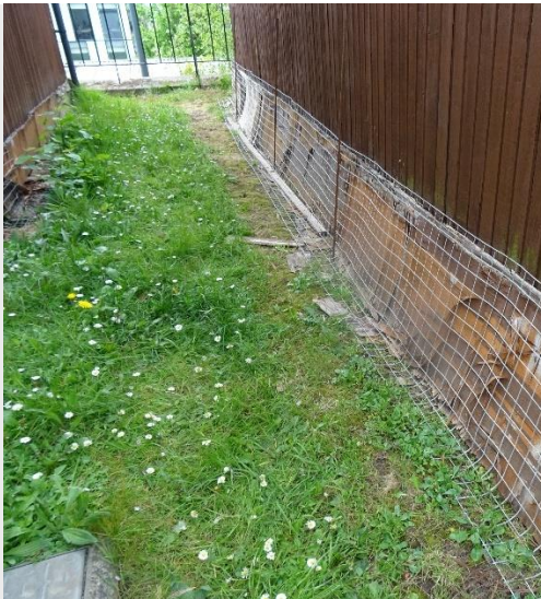
Photograph 3. The area under the buildings has been sealed against animal ingress
