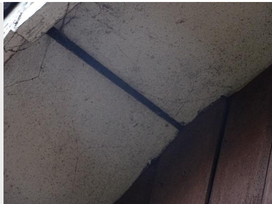
Photo 11. West flank wall gable apex
