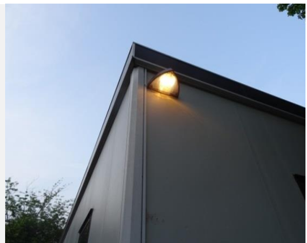
Photograph 4. Indicating the lights that exist at each corner of the building
