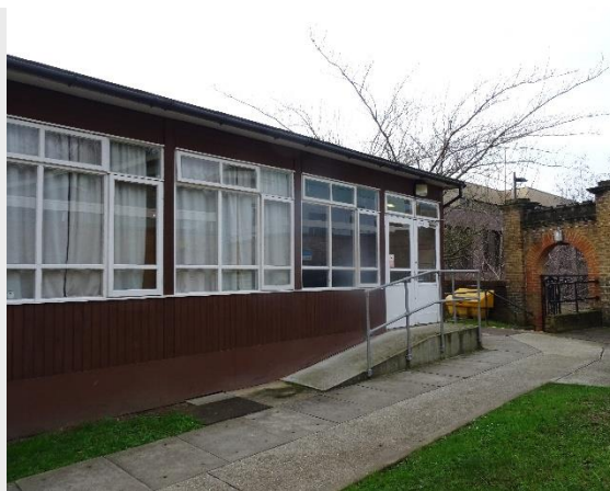
Photograph 7 Hut 2 with access ramp
