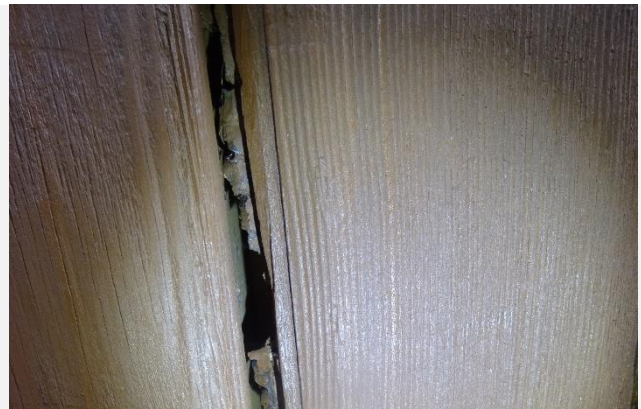
Photo 12. Cladding on west elevation
