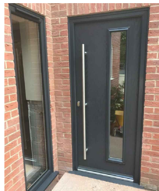
ALL JOINERY TO BE ALUMINIUM FINISHED IN BLACK GREY RAL 7021
