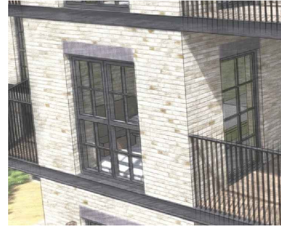
MILD STEEL FEATURE BEAMS AND POWDER COATED METAL GUARDING/HANDRAIL COLOUR - BLACK GREY RAL 7021
