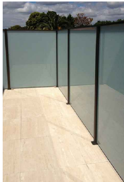
FROSTED GLASS PRIVACY SCREEN WITH TOP SET AT 1.8M ABOVE FINISHED TERRACE
