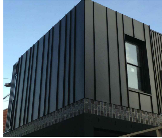
STANDING SEAM ZINC CLADDING IN BLACK GREY RAL 7021
