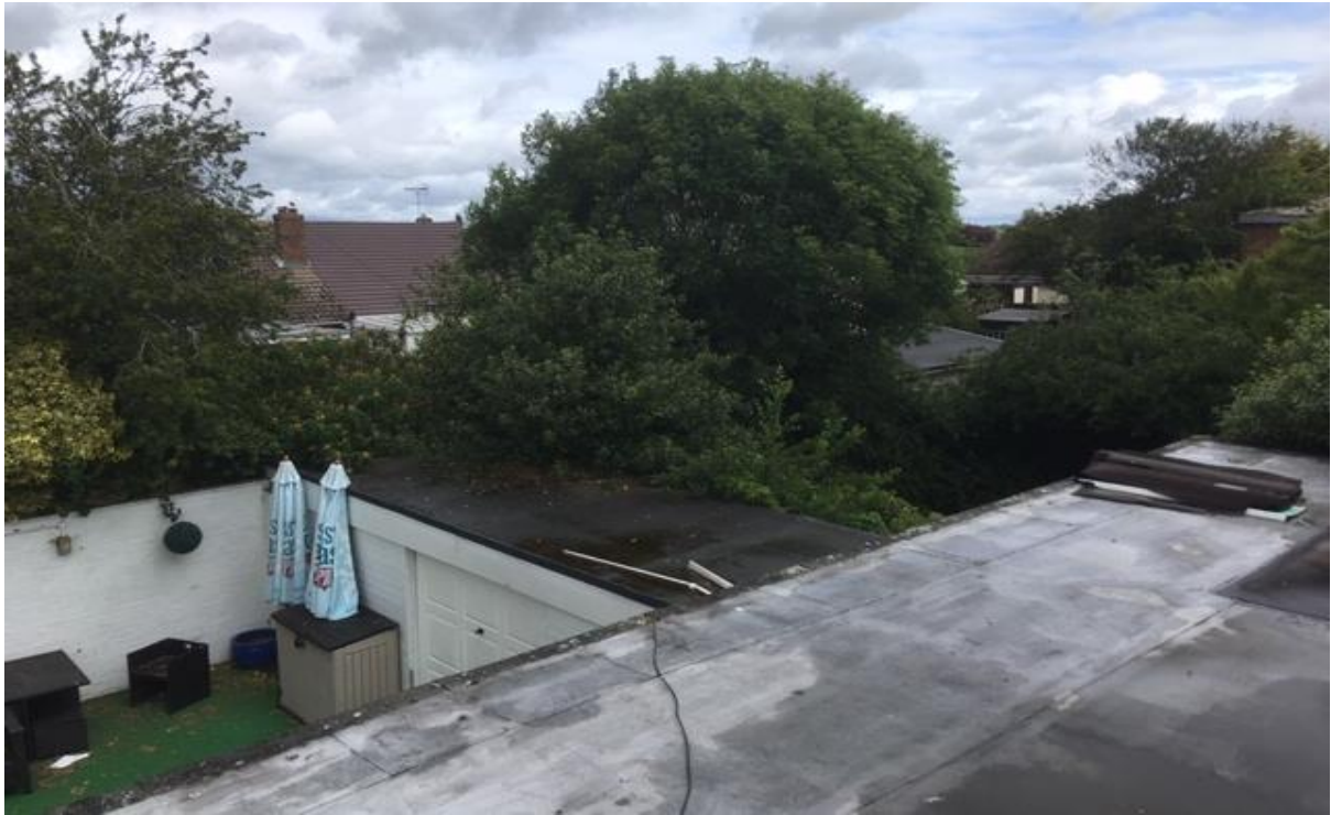
3 – View of Colchester Road properties from Function Room Roof
