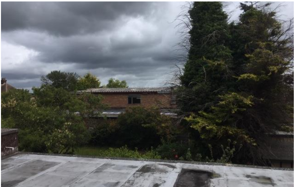
4 – View of Industrial unit from Function Room roof
