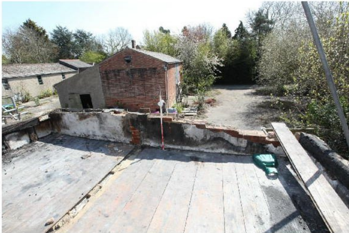
Illus. 34. The south-eastern gable of 19 th century brickwork with the farm yard and mid-19 th century brick threshing barn beyond. The gable and south-western wall may have been rebuilt in brick as part of the same site refurbishment that included the barn. Most farm yards in the region adjoined service rather than parlour gables.
