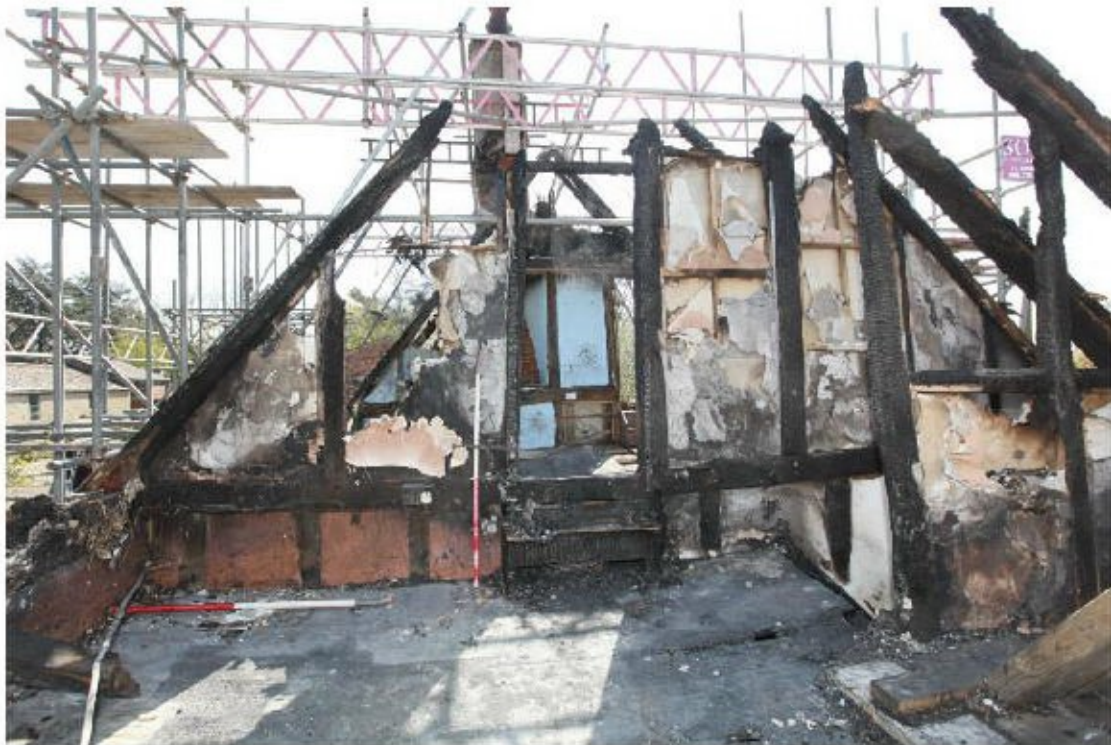
Illus. 25. The chamber above the probable parlour from its gable to the north-west showing the fully framed partition adjoining the central hall chamber. The jamb of the original ground-floor door lies close to the storey post on the left with a pegged short stud above the lintel and the first-floor door is an insertion between to original studs. The floorboards consist of recent softwood throughout the upper storey with no evidence of earlier boards beneath.
