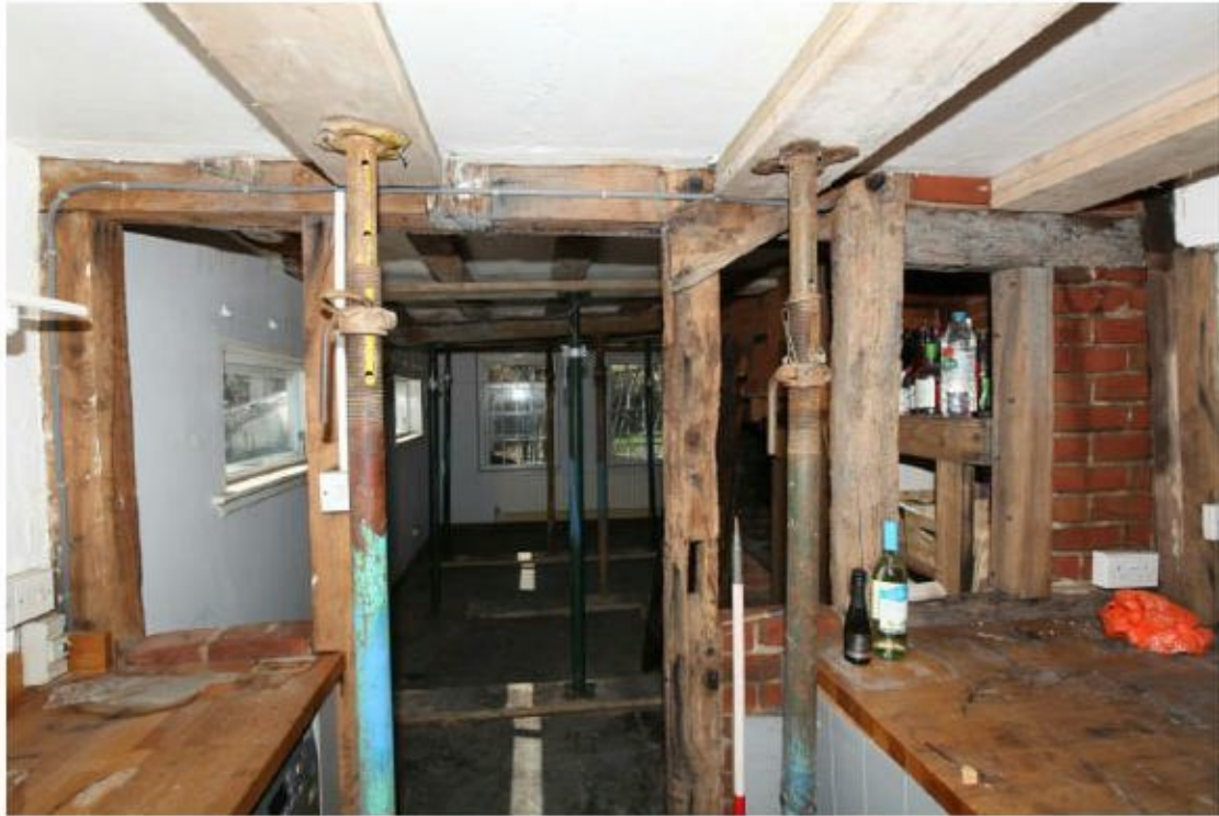
Illus. 21. The exterior of the parlour's rear wall from the lean-to kitchen extension showing two original truncated studs above the modern false studs on the left and a truncated original externally trenched wall brace against the central stud. The original window jamb and lintel are visible on the right.
