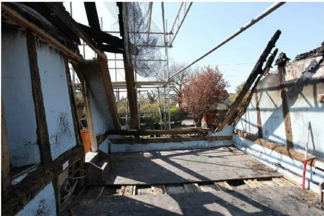
Illus. 28. The central hall chamber showing the largely intact, fully framed partitions of the probable parlour bay and service bays to the right and left respectively. The modern softwood floorboards are laid directly onto the ground-floor ceiling joists with plasterboard infill. The south-western roof-plate in the rear has been entirely renewed in modern oak.
