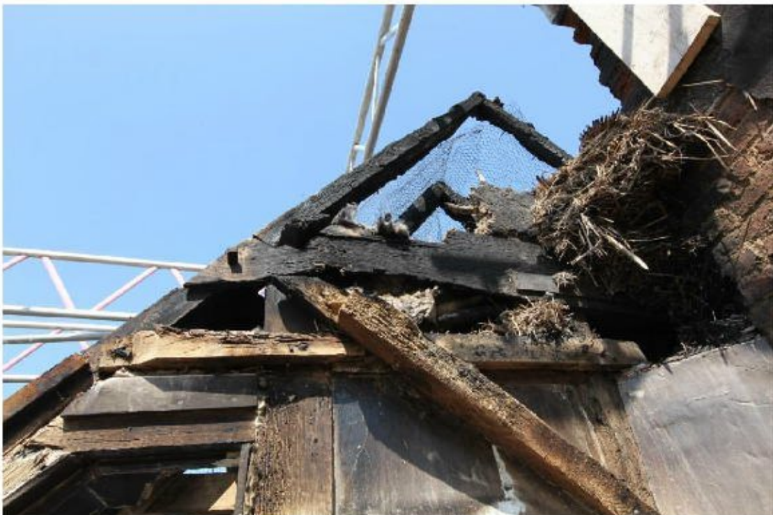
Illus. 32. A detail of the single remaining truss of the probably original clasped-purlin roof structure with pegged collars but no evidence of wind-braces (to the left of the chimney in illustration 31). Despite the lack of wind-braces this roof is consistent with the late-16 th century date indicated by the wall framing, particularly as the collar is dovetailed rather than simply lapped. The nailed lower collars held the later ceiling.
