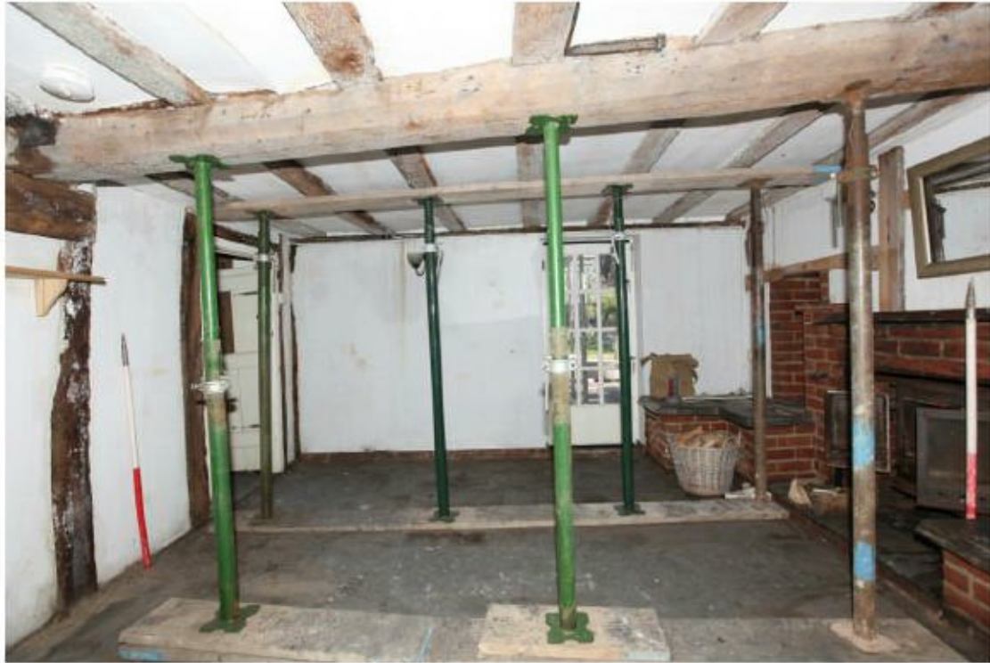
Illus. 5. The central hall from the south-west showing the rendered rear (north-eastern) wall with the modern fireplace in the original chimney on the right and the ostensible 'high end' wall to the left. The complete 16 th or early-17 th century ceiling has been inserted into a former open hall.
