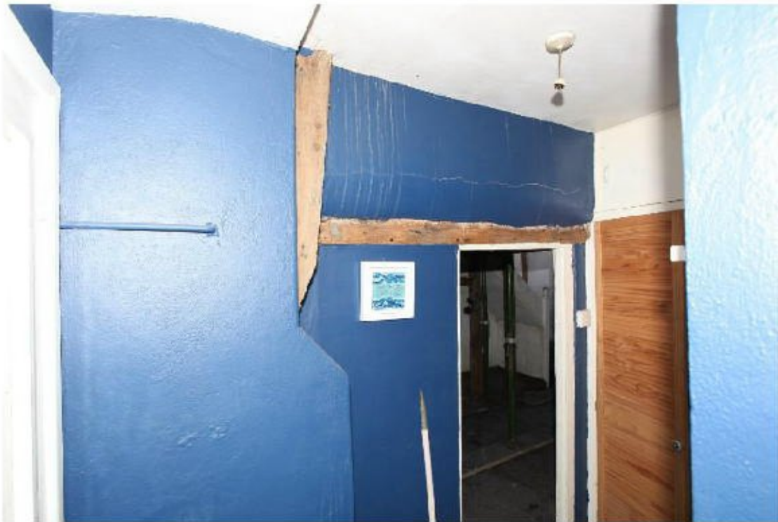
Illus. 14. The northern corner post of the original structure from its later extension showing the ceiling rail or clamp of the service gable from which the lower studs have been removed. The jowled post contained a double-pegged mortice for a descending externally trenched wall brace.
