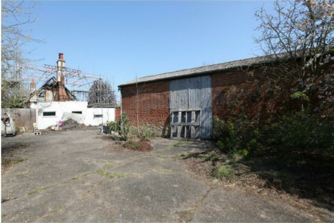
Illus. 3. The cottage from its former farm yard to the south-east showing the late-20 th century horizontal windows of its 19 th century gable of painted brick with the mid-19 th century threshing barn on the right. The latter's doors are respected by the bonding.
