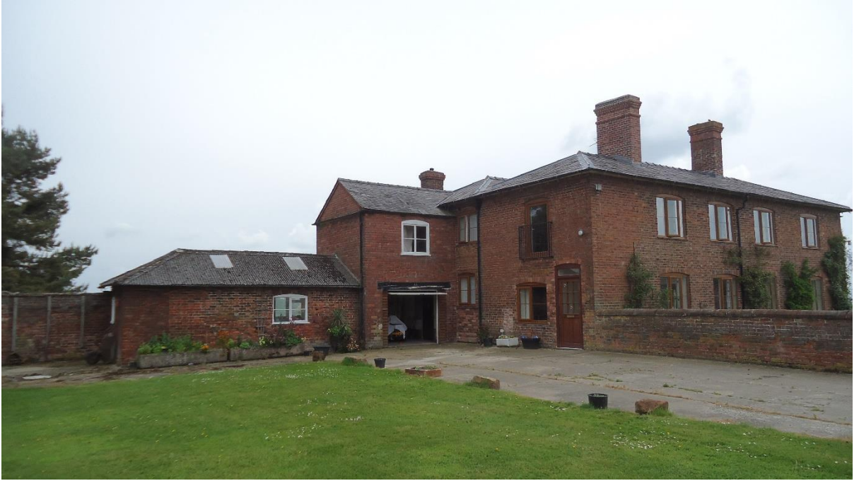
Photograph 3 West elevation of house.
