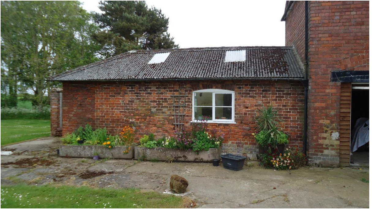
Photograph 1 Existing west elevation
