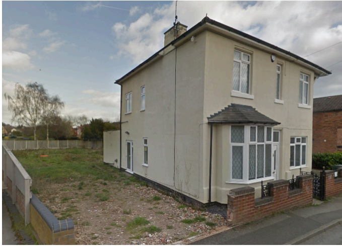
6.1 The existing main two-storey building.
