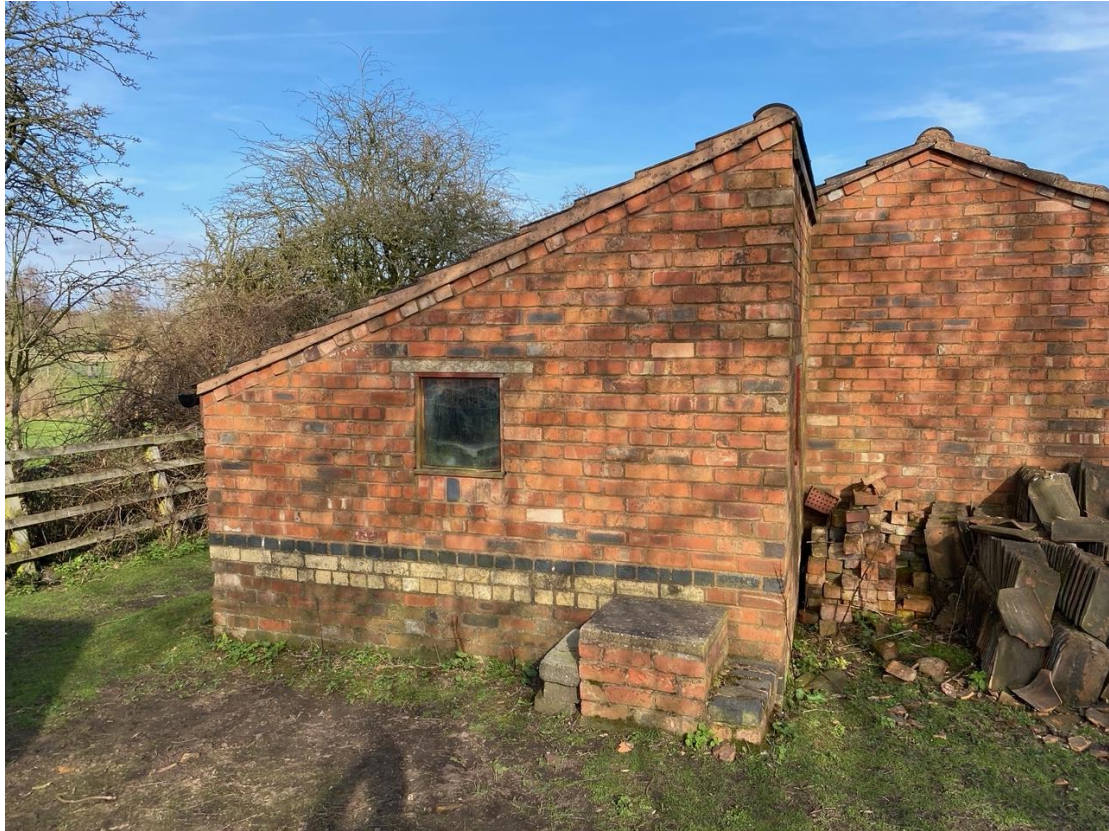
3. Left-hand elevation (tack room)
