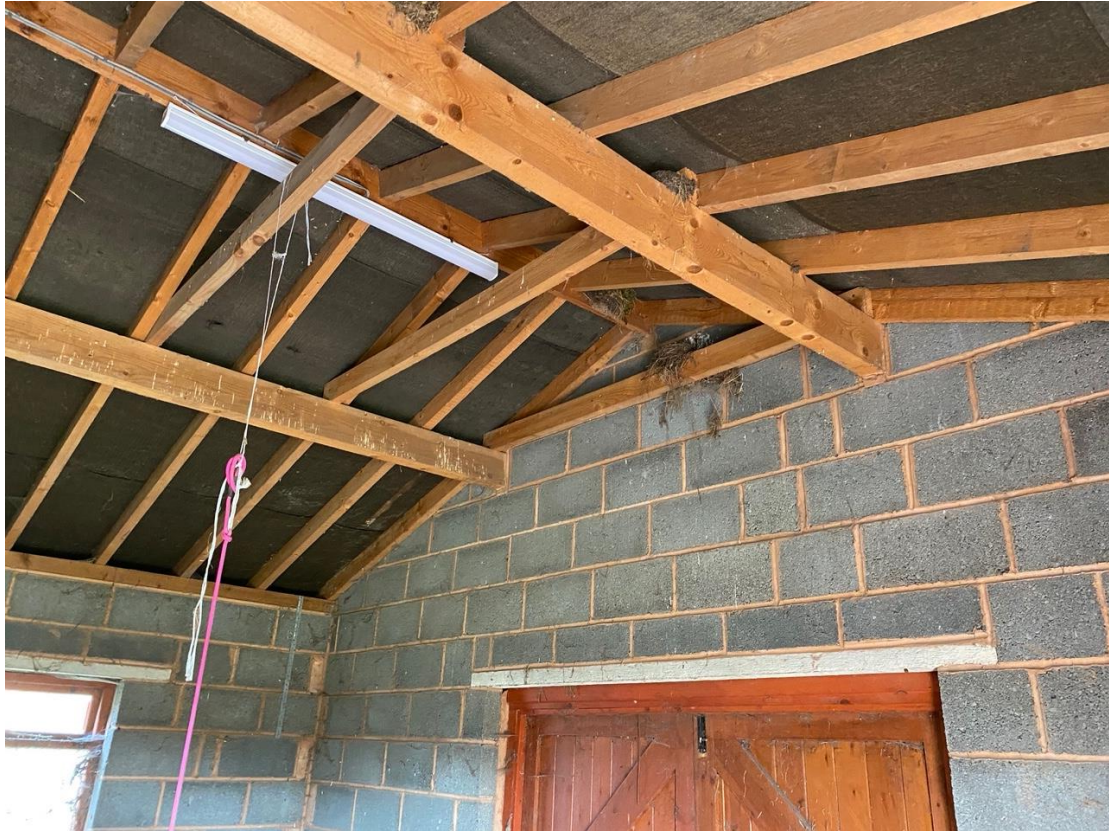
11. Internal view of right-hand gable wall
