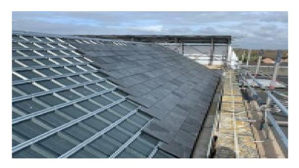
Kingspan Nulok Slate Roofing System (slate grey) Please refer to the separate Kingspan Manufacturer Sheet submitted as part of the NMA.
