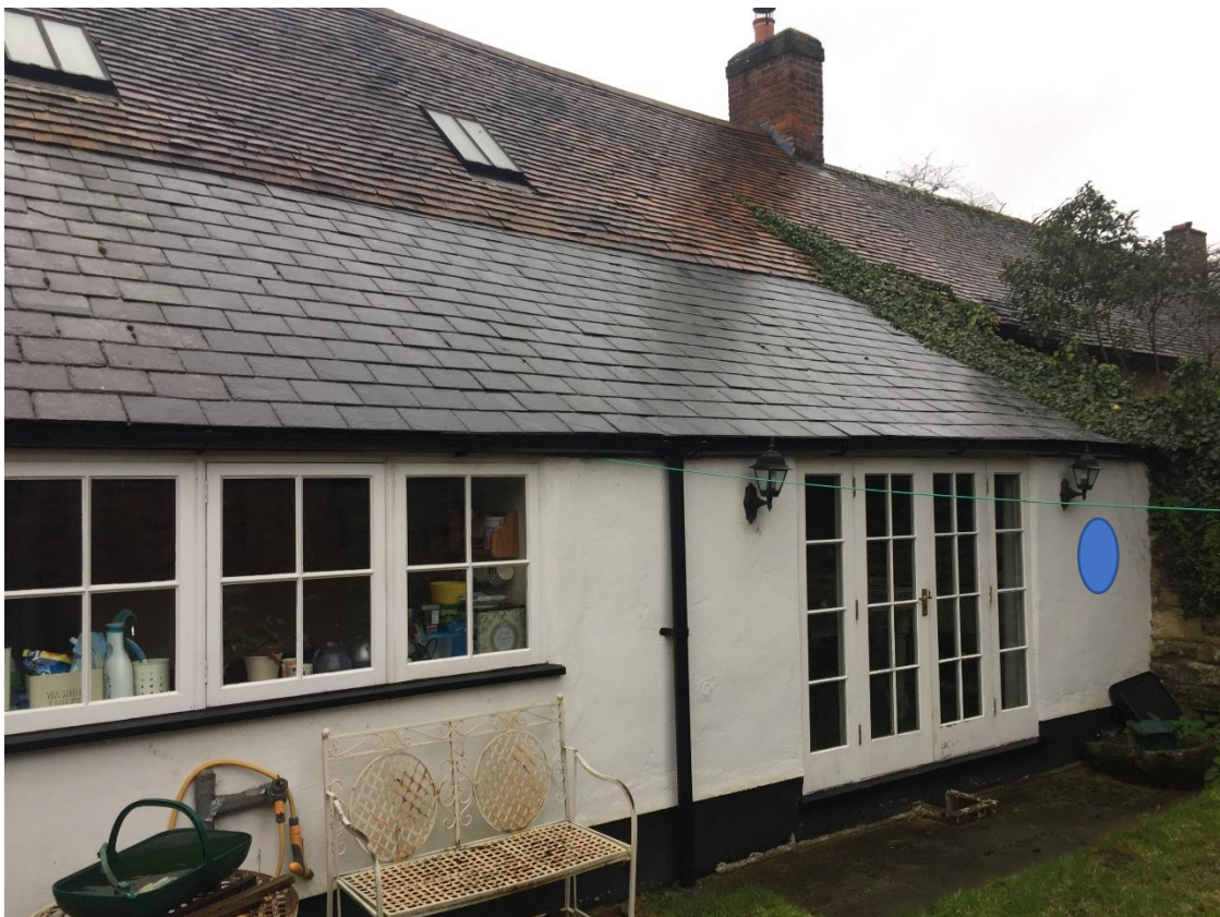
The rear extension – looking west
