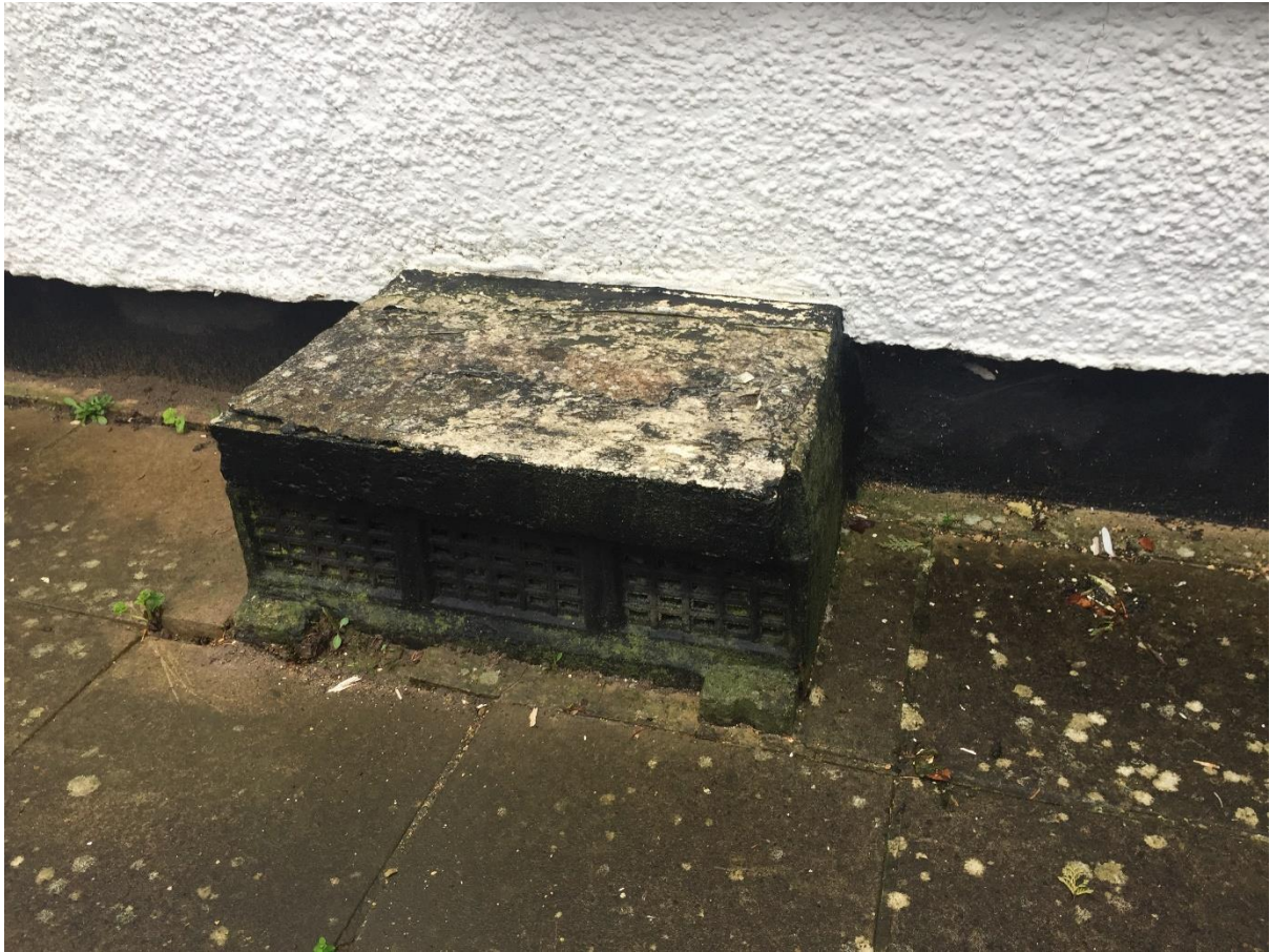
The cellar ventilation cover
