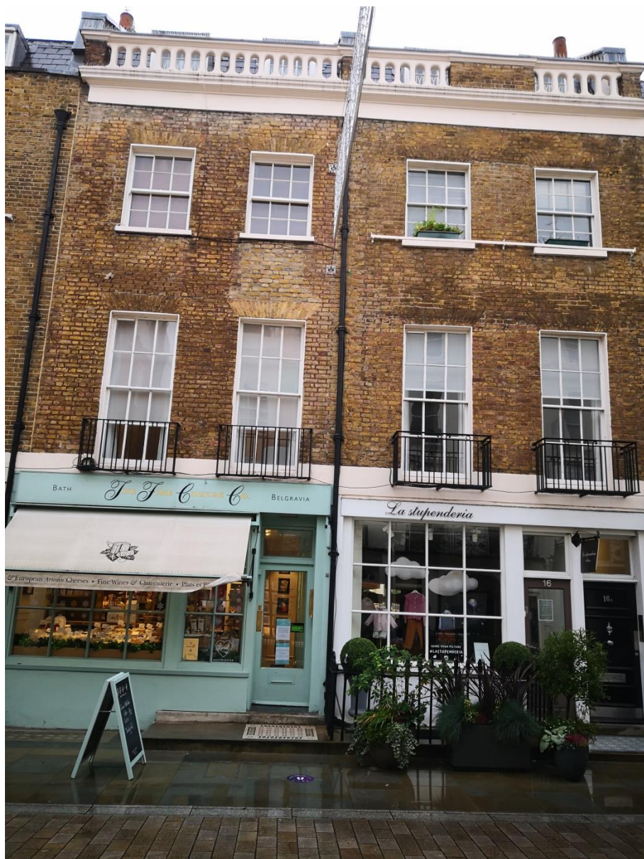
Front of Nos. 16 (right) and 17 (left), which remain unaltered in this application
