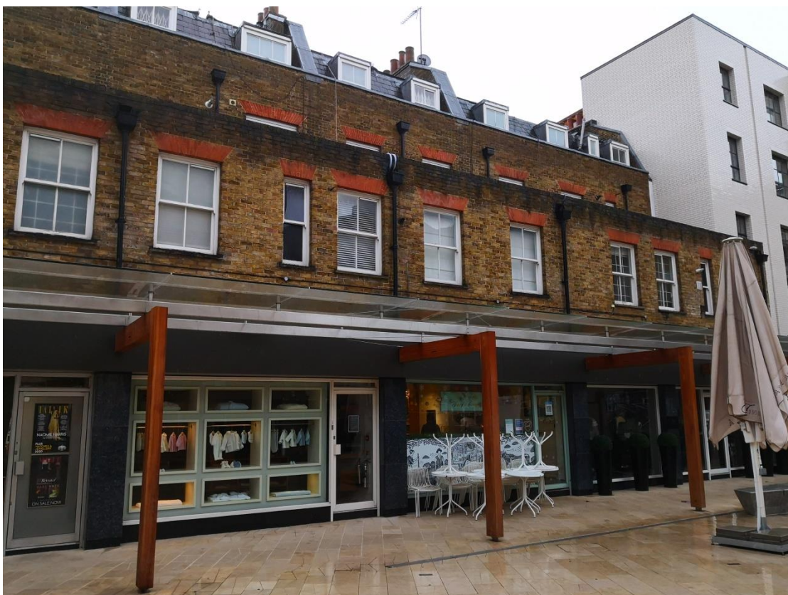
Rear of Nos. 16 (left) and 17 (right) seen from Halkin Arcade, showing 1970s two storey extension, further altered on ground floor with canopy. Photograph taken from standing in area outside designated Conservation Area.
