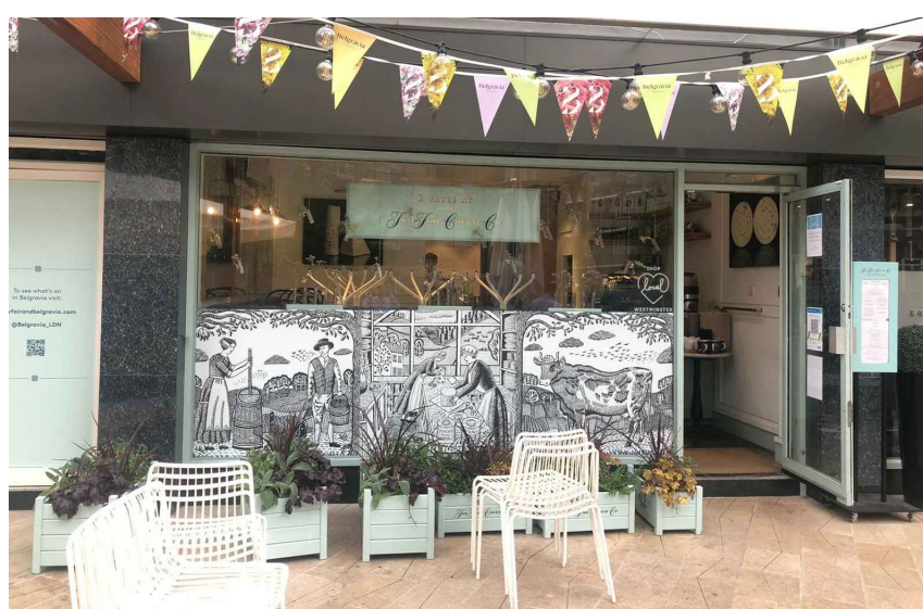
EXISTING SHOPFRONT UNIT 17
