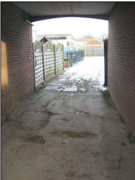
03 - Archway leading to rear access
