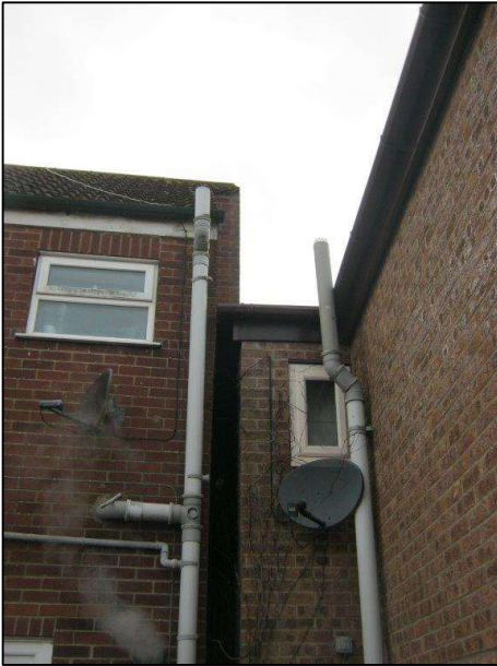
05 – Void to northern boundary
