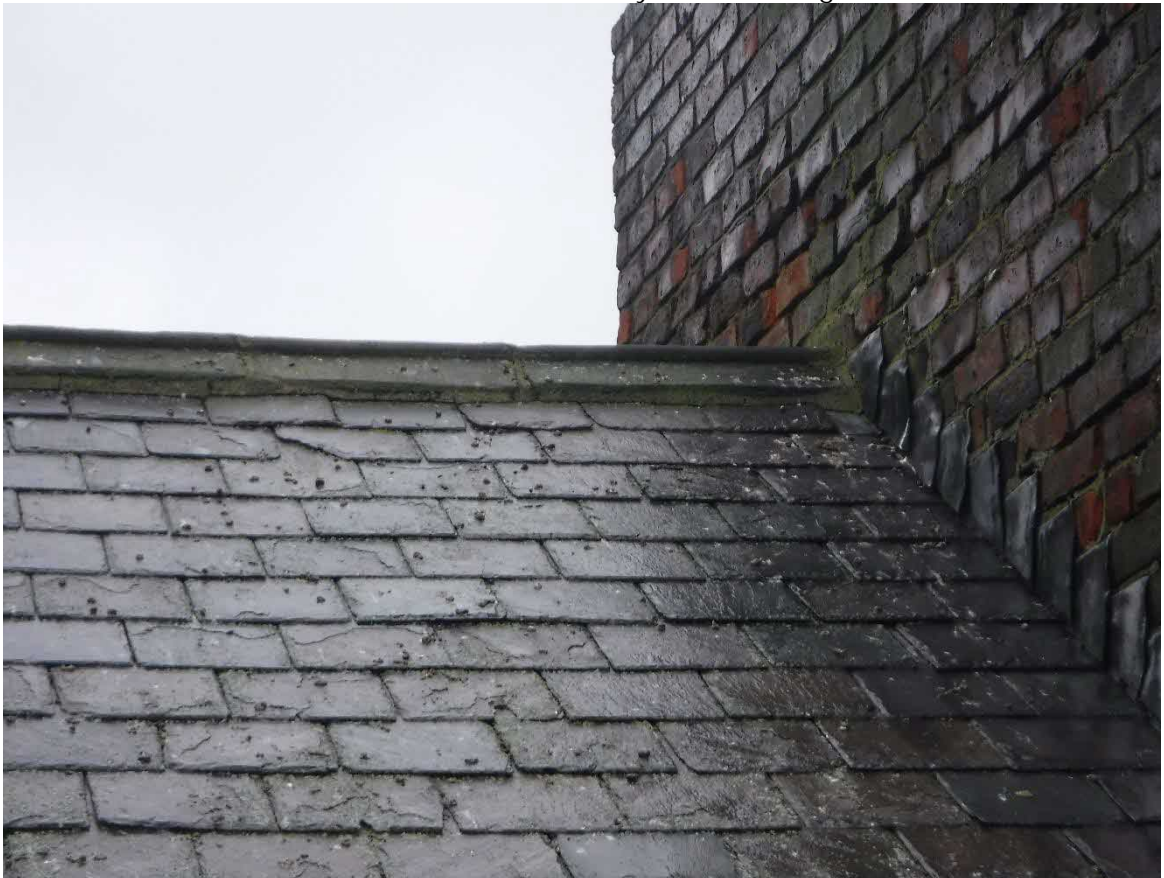
Photo 8 – Front Elevation – Central chimney stack and ridge to LHS of stack
