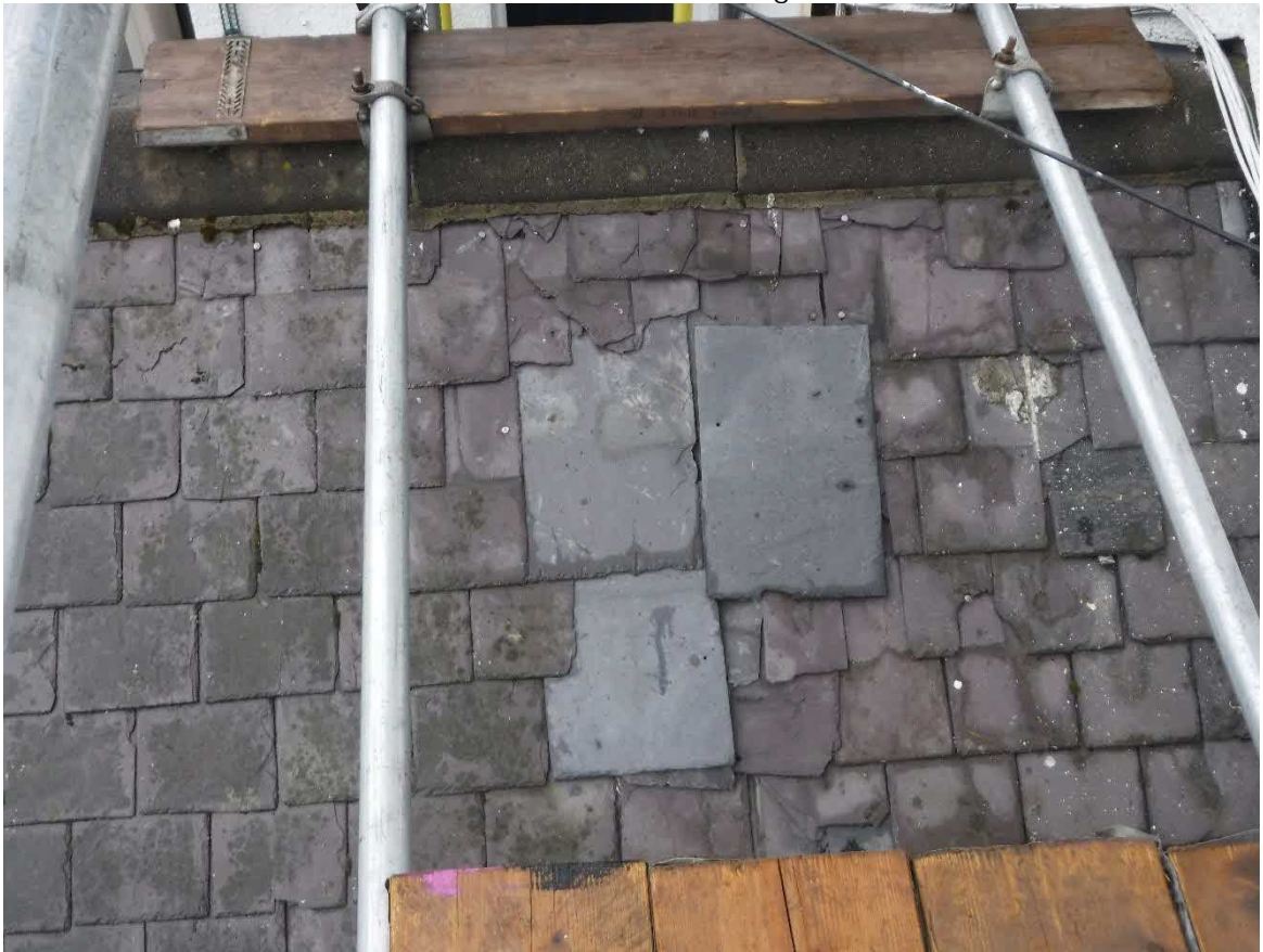
Photo 20 – Rear Elevation – Roof covering of rear off-shoot
