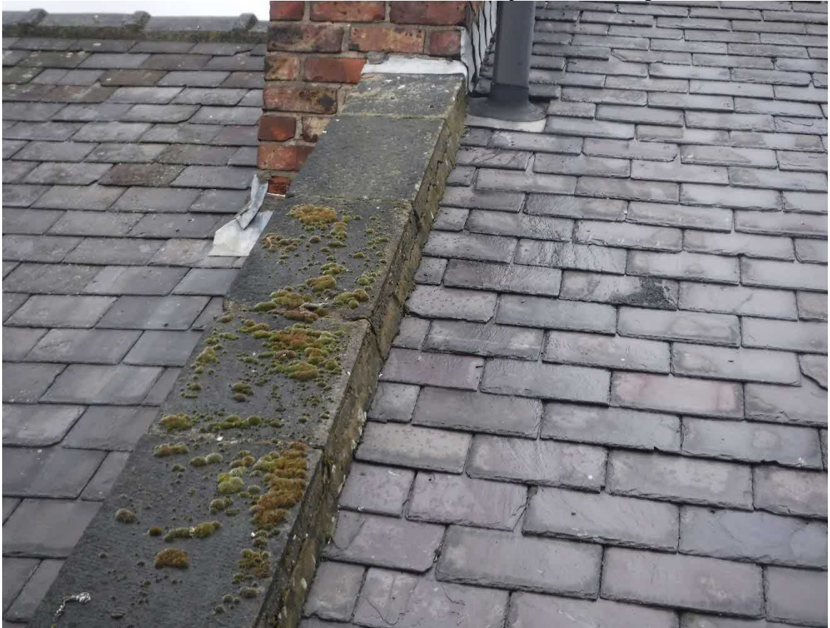
Photo 33 – Rear Elevation – LHS chimney stack and verge
