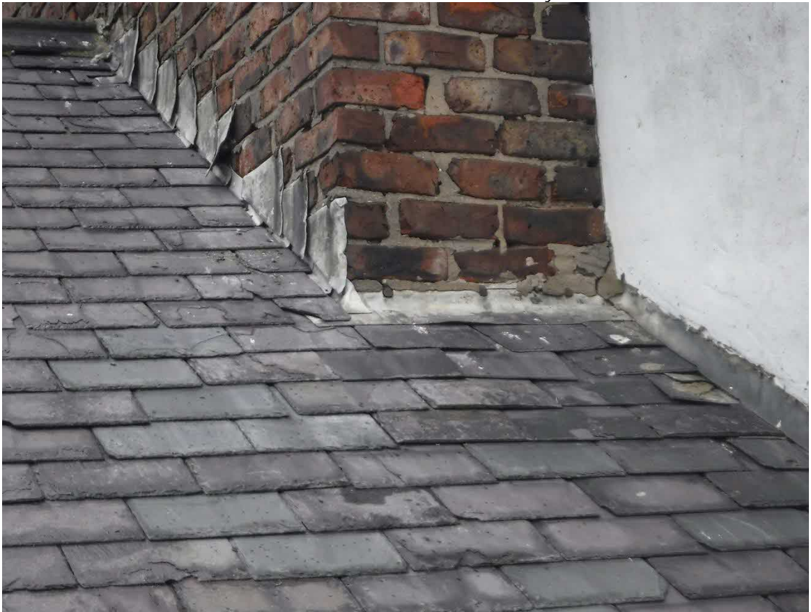
Photo 30 – Rear Elevation – RHS chimney stack
