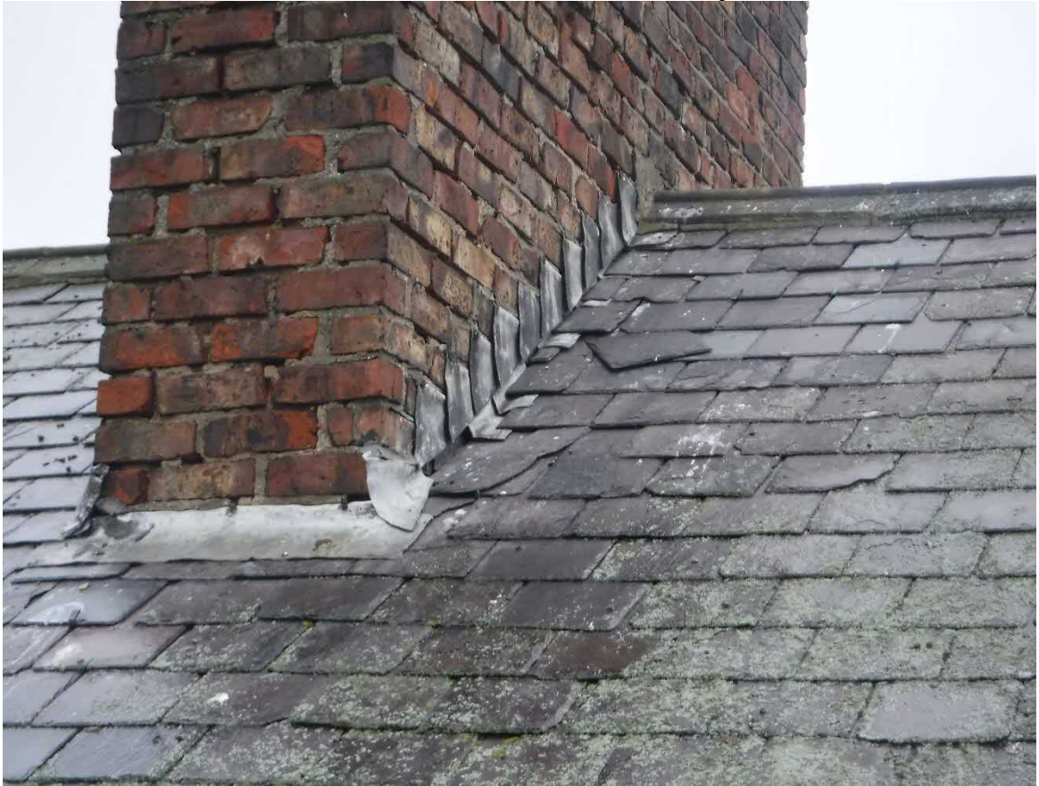
Photo 13 – Front Elevation – Central chimney stack
