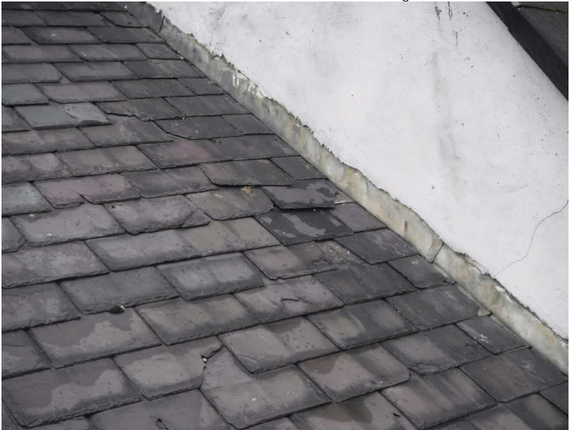
Photo 34 – Rear Elevation – Roof covering
