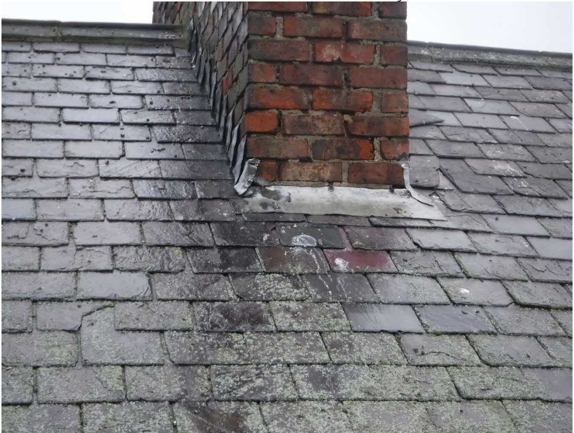
Photo 10 – Front Elevation – Central chimney stack
