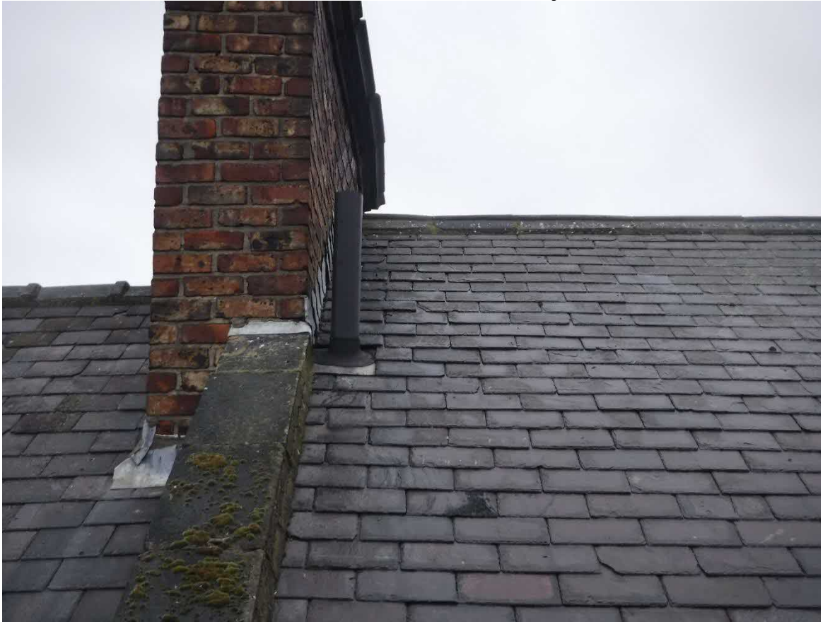
Photo 23 – Rear Elevation – LHS chimney stack
