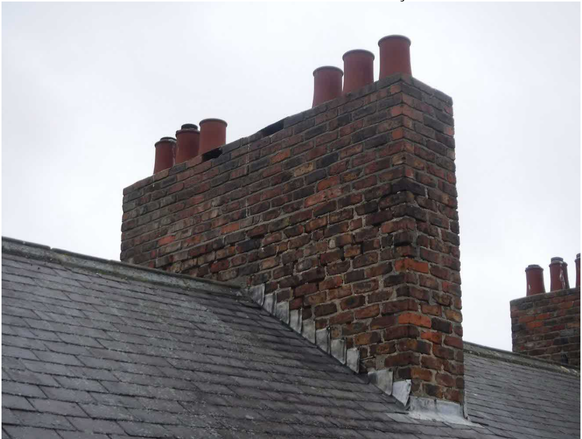
Photo 24 – Rear Elevation – Central chimney stack
