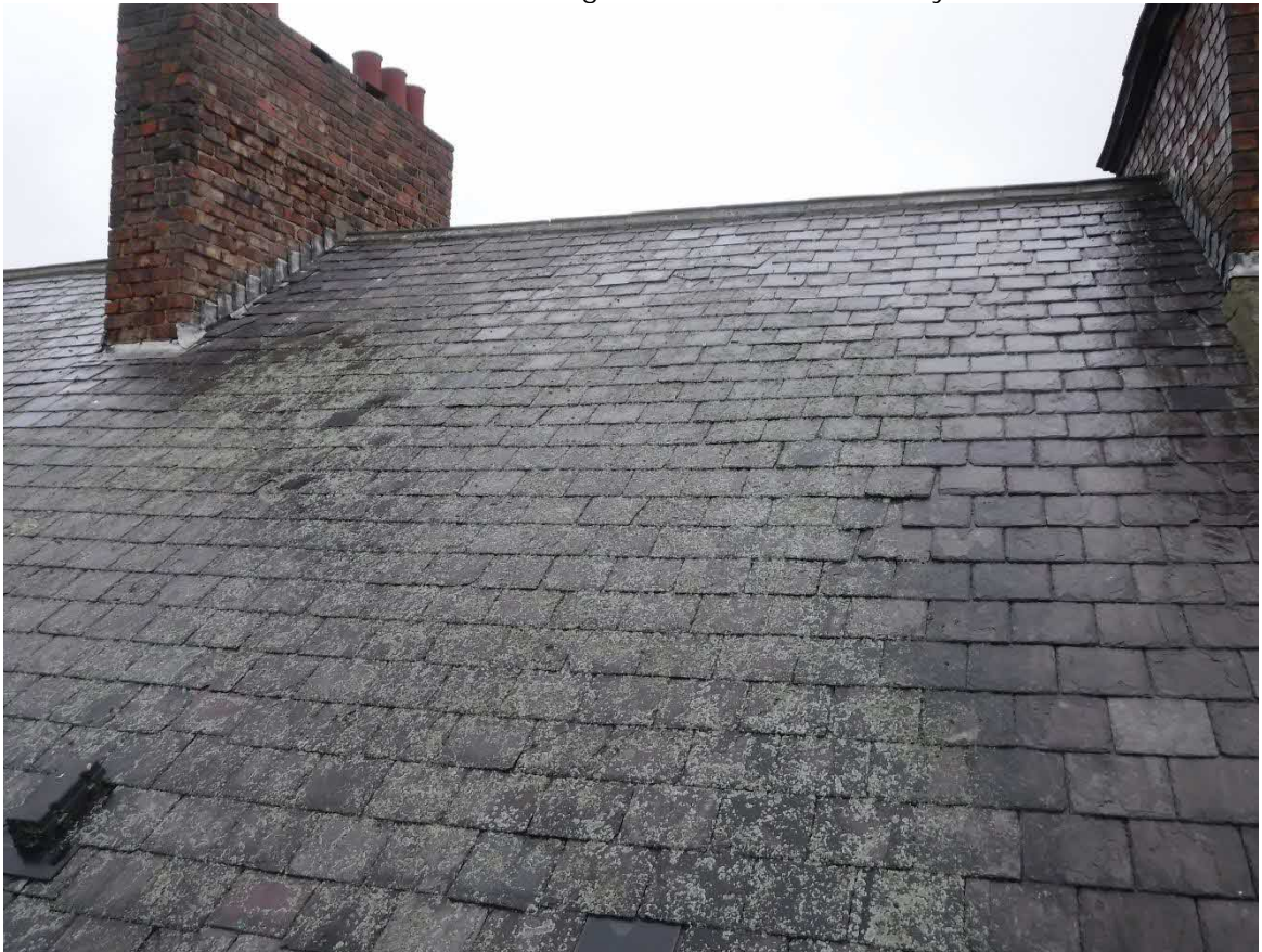
Photo 16 – Front Elevation – Roof covering between central chimney stack and RHS stack
