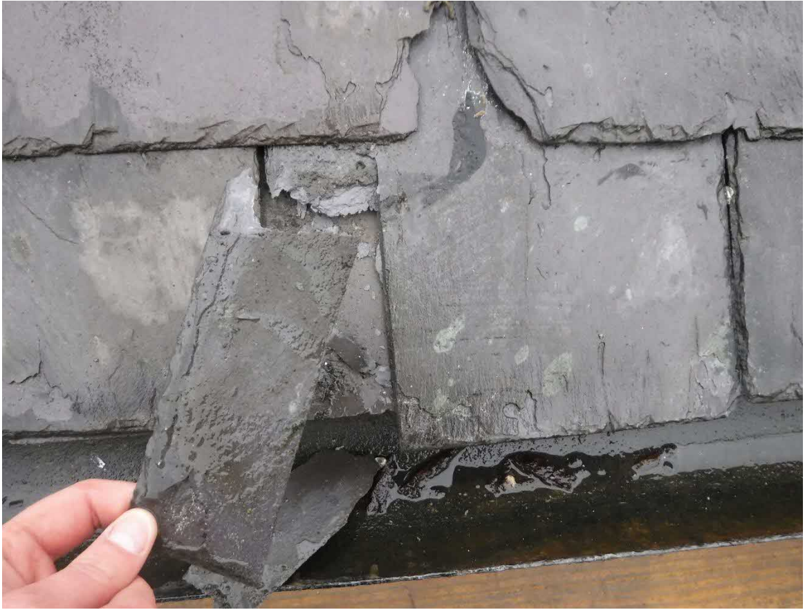
Photo 31 – Rear Elevation – Roof tile
