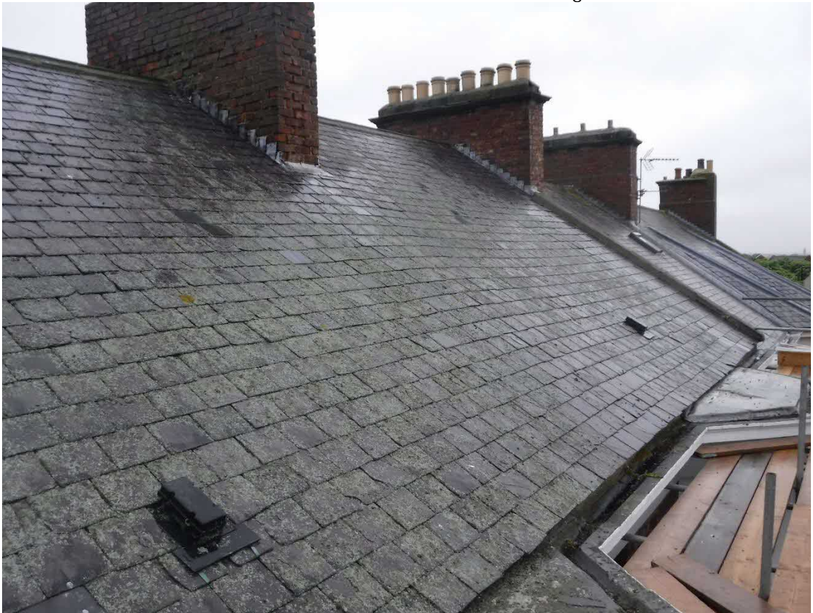
Photo 2 – Front Elevation – Roof covering
