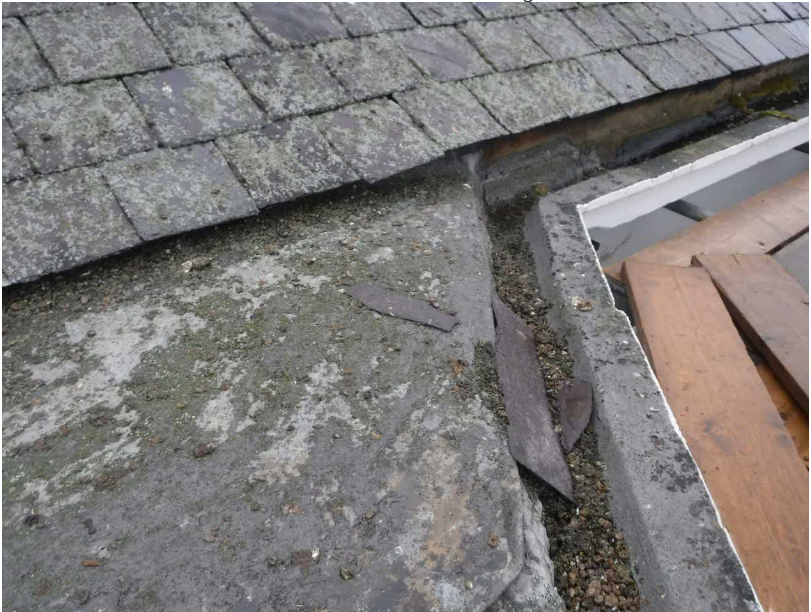
Photo 4 – Front Elevation – Finlock gutters
