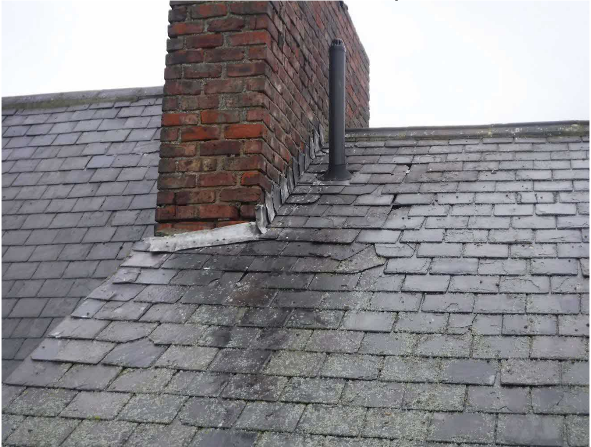
Photo 5 – Front Elevation – LHS chimney stack
