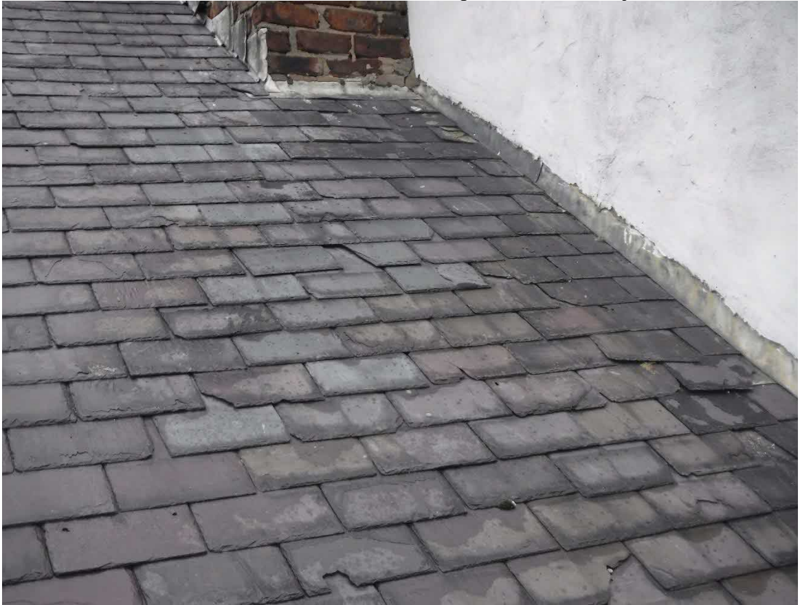
Photo 29 – Rear Elevation – Roof covering near RHS chimney stack
