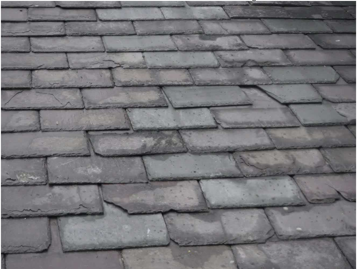
Photo 32 – Rear Elevation – Roof covering
