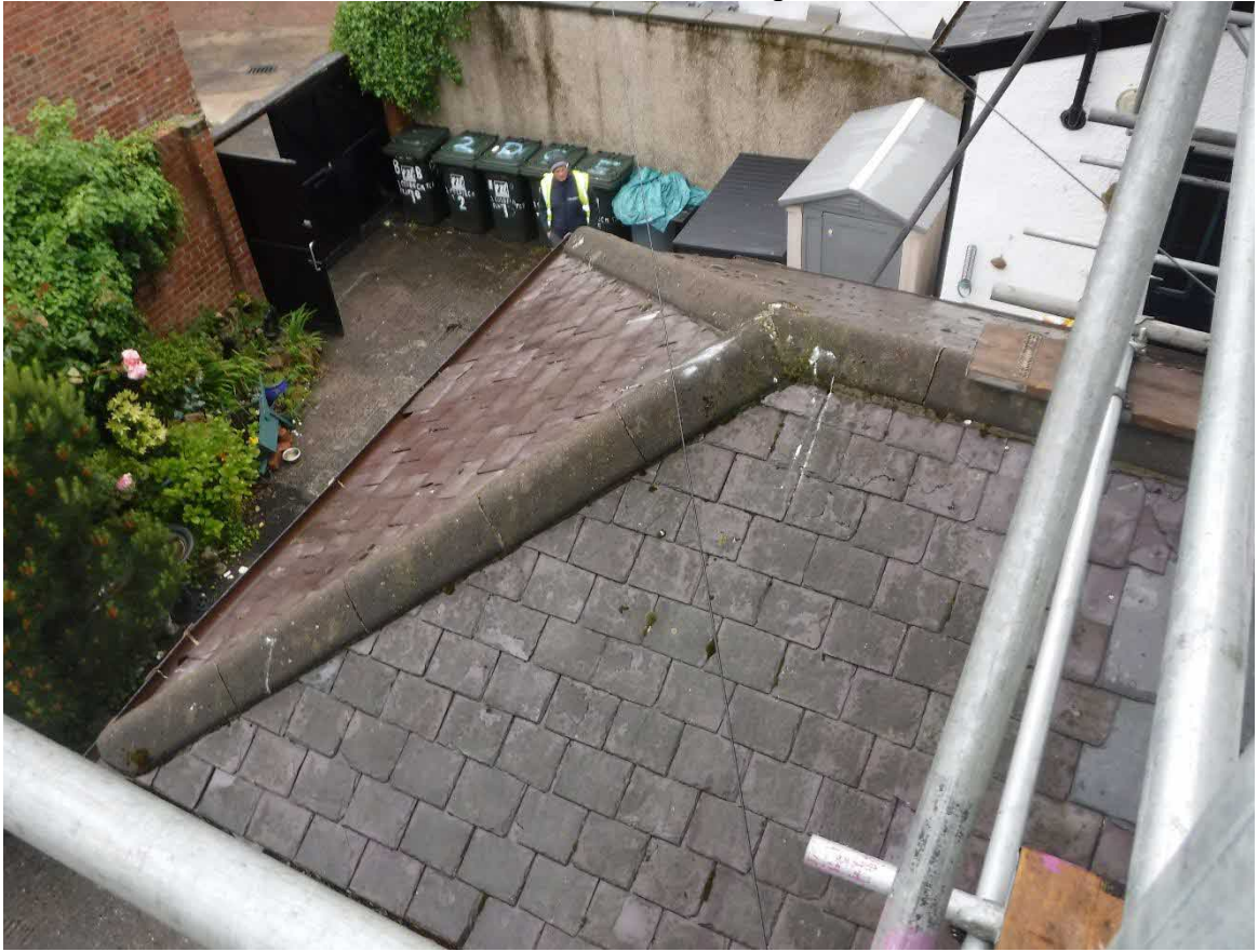
Photo 19 – Rear Elevation – Roof covering of rear off-shoot
