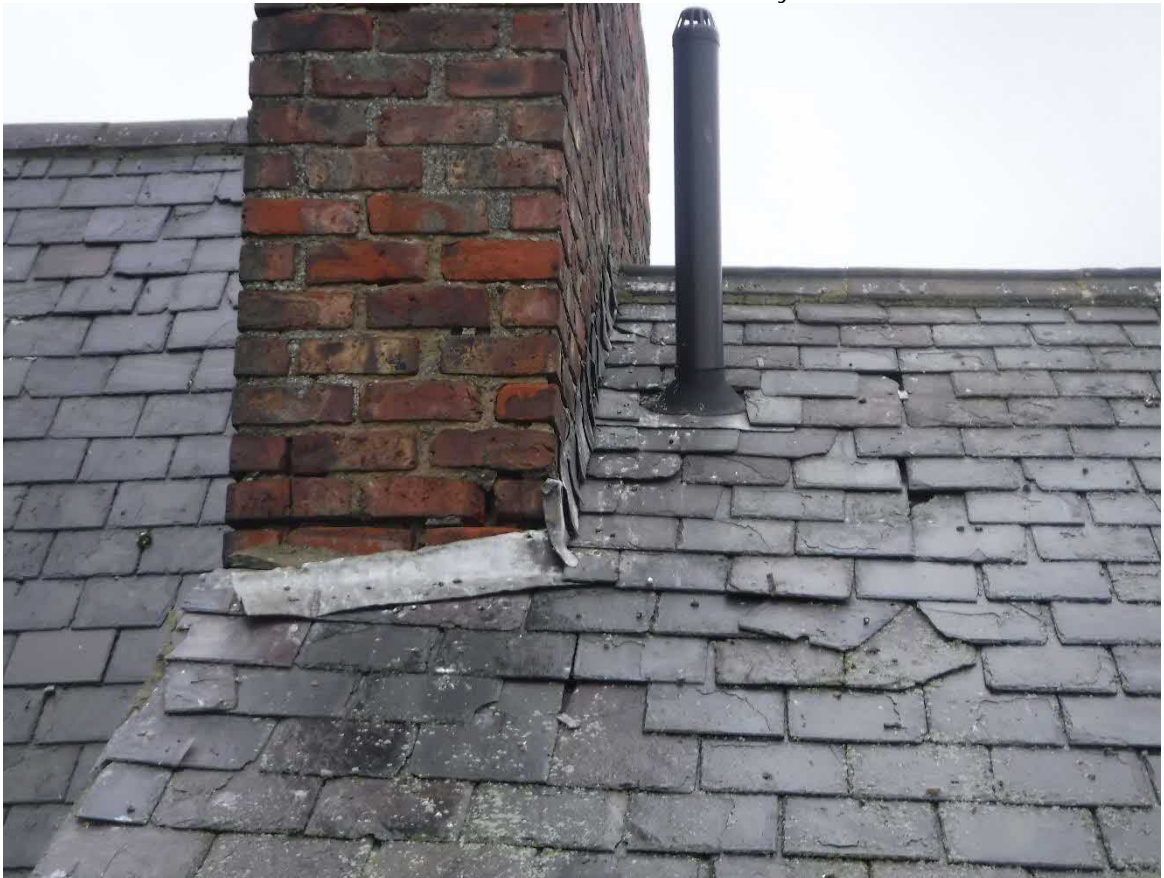
Photo 6 – Front Elevation – LHS chimney stack
