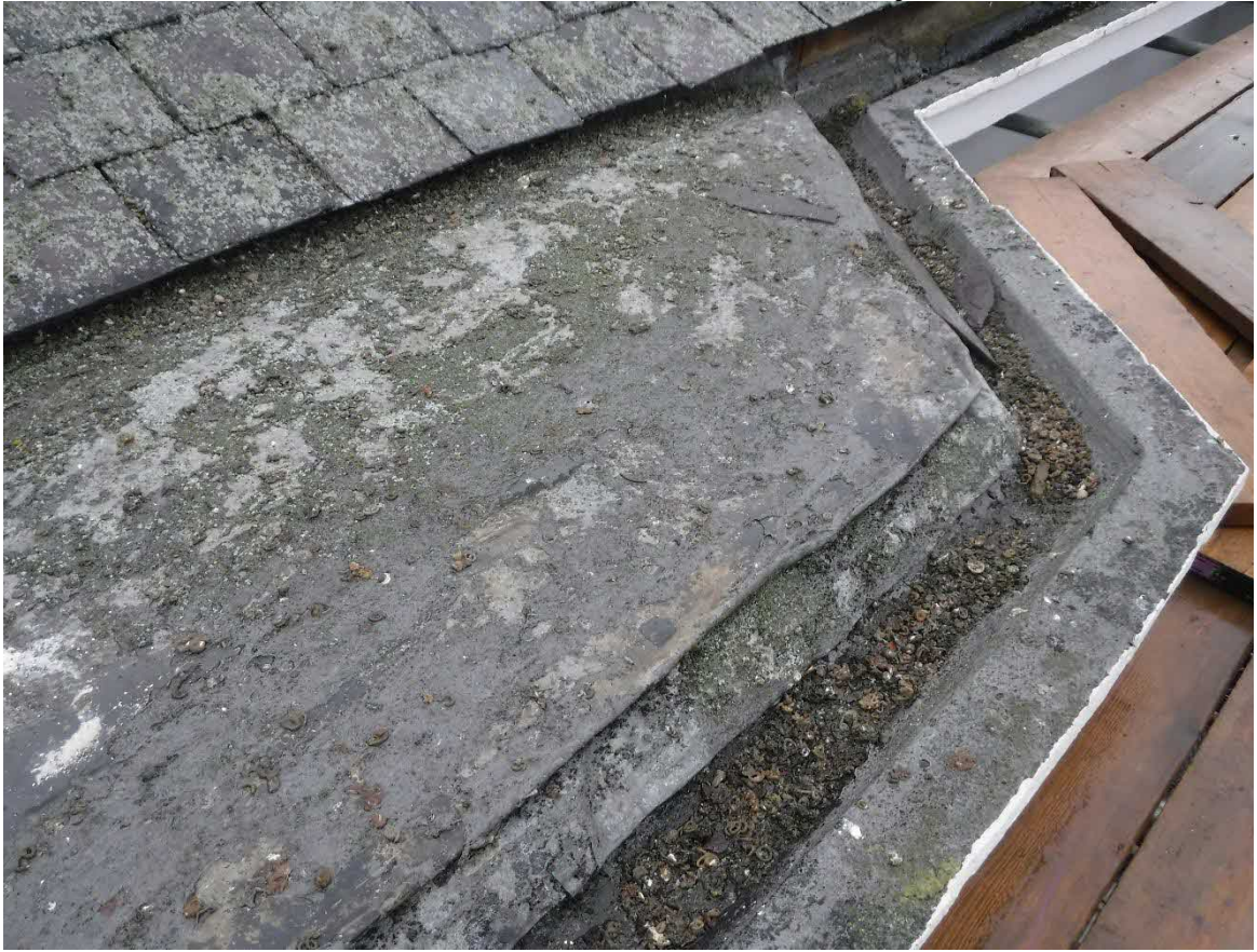
Photo 4 – Front Elevation – Finlock gutters
