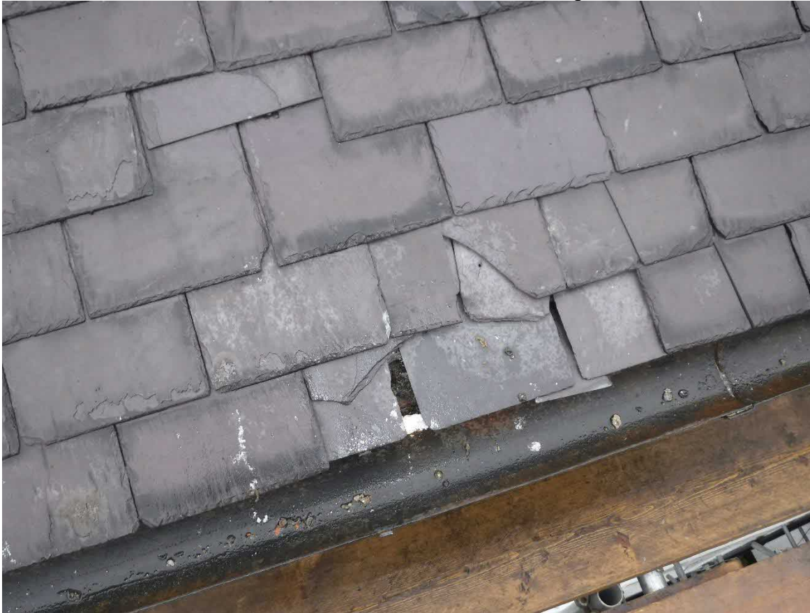
Photo 28 – Rear Elevation – Roof covering
