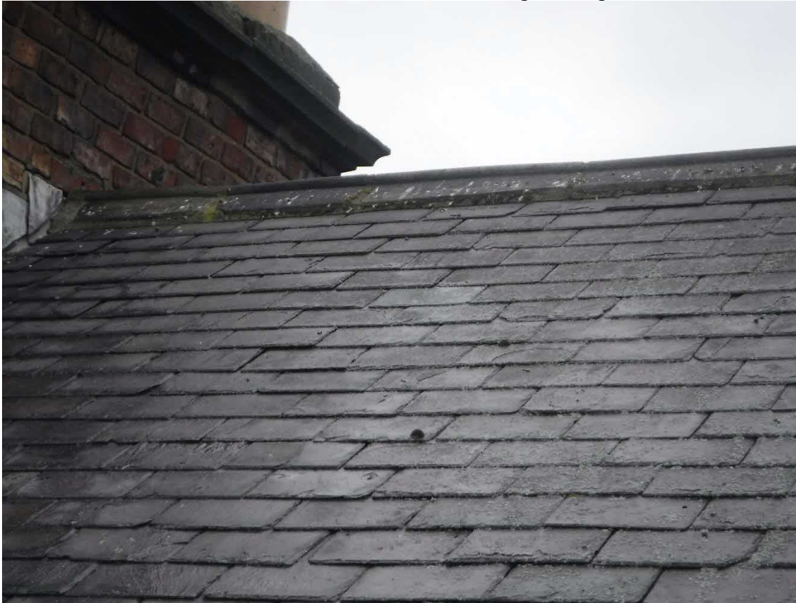
Photo 27 – Rear Elevation – Roof covering and ridge
