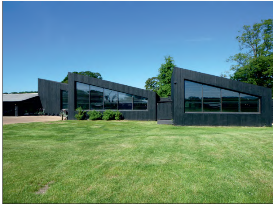
Photograph 1: Showing the front of the existing gym structure.
