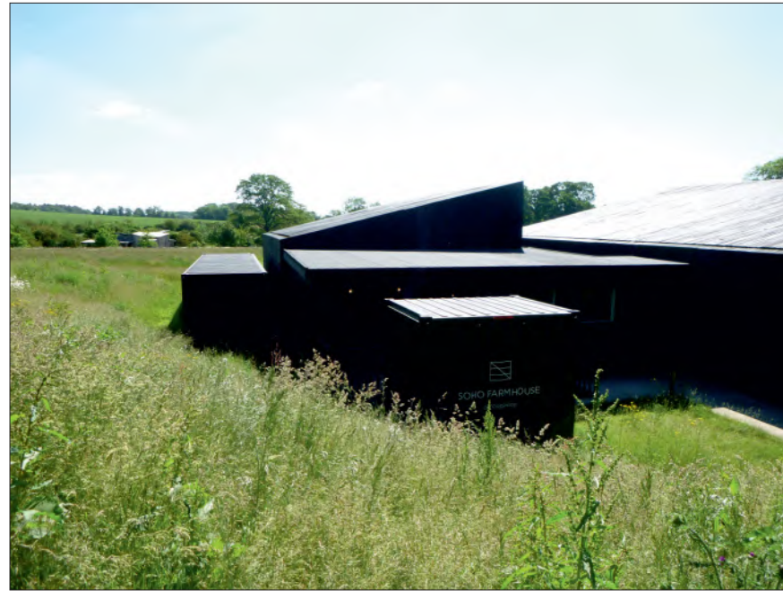
Photograph 2: Showing the rear of the existing gym structure.
